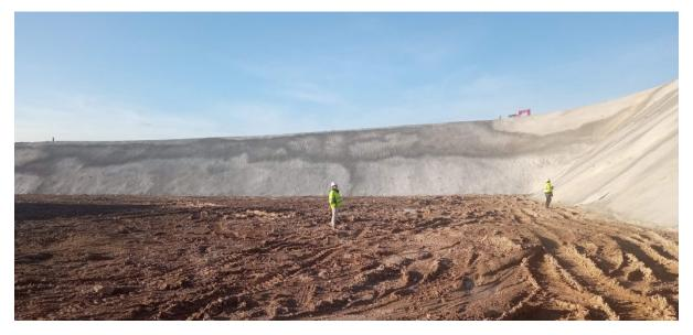
FIGURE 1. OVERVIEW OF THE BOX CUT AND SURFACE DRAINAGES FROM THE TEMPORARY EMBANKMENT
