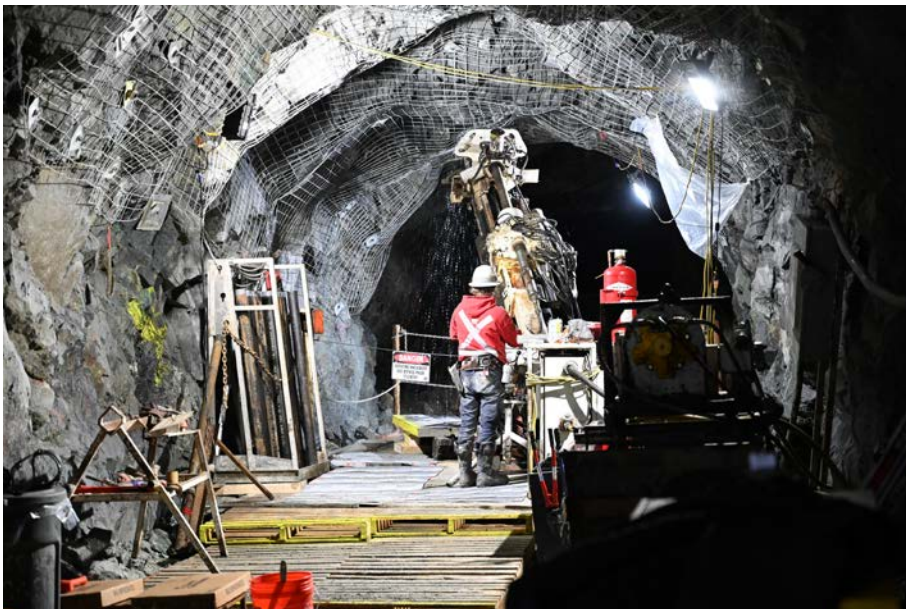
Photo 1 – Underground drilling at Oracle Ridge.
