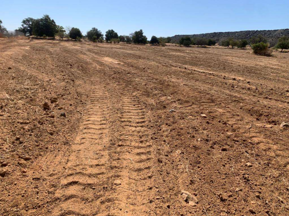
Leveling of land previously disturbed by artisanal gold mining in preparations for rehabilitation during the next rainy season
