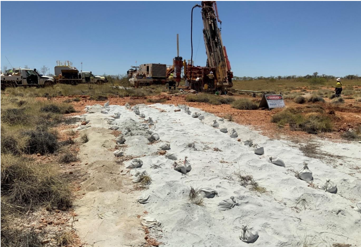
Figure 8 - MBRC047 Talga – Mollyella drill pad November 2022 with extensive intersections of multiple stacked Pegmatites.
