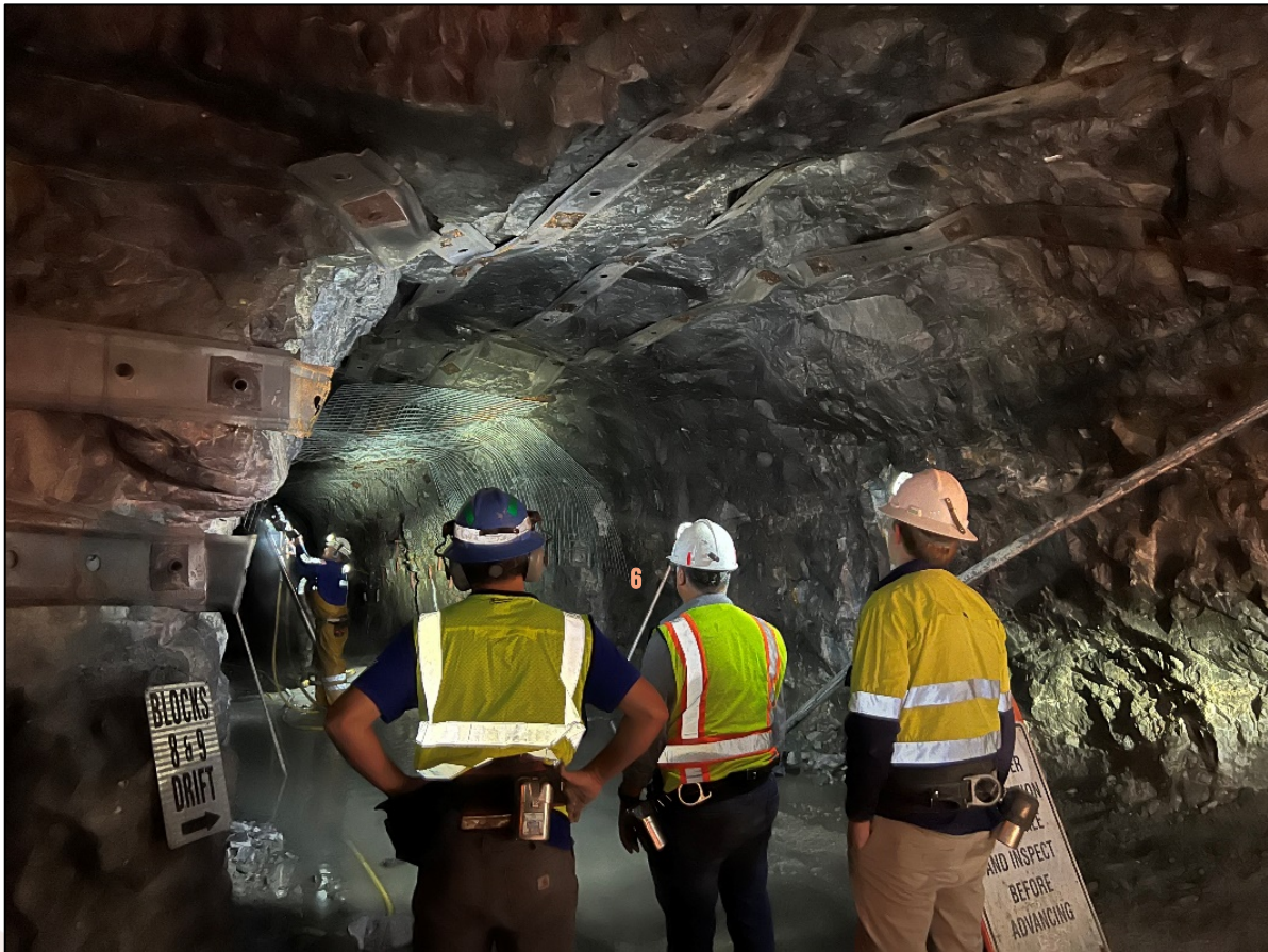
Photo 1 - Installation of ground support
