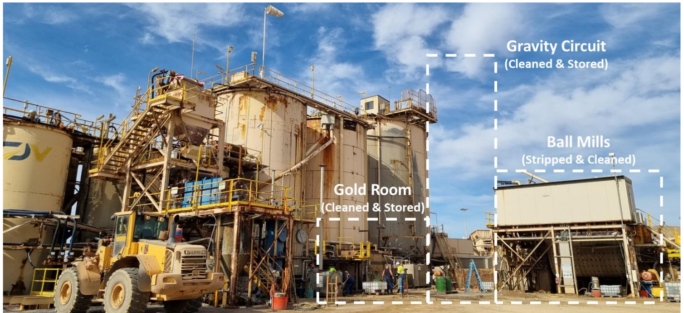
Figure 6 – Central Gawler Mill with Gravity Circuit & Gold Room Removed 6
