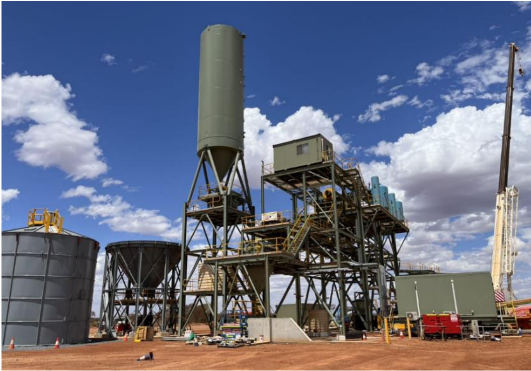
Figure 10 – Paste plant structural steel being erected (December 2022).
