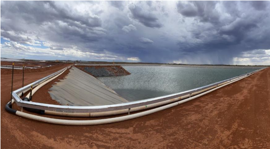
Figure 14 – Tailings storage facility TSF (December 2022).
