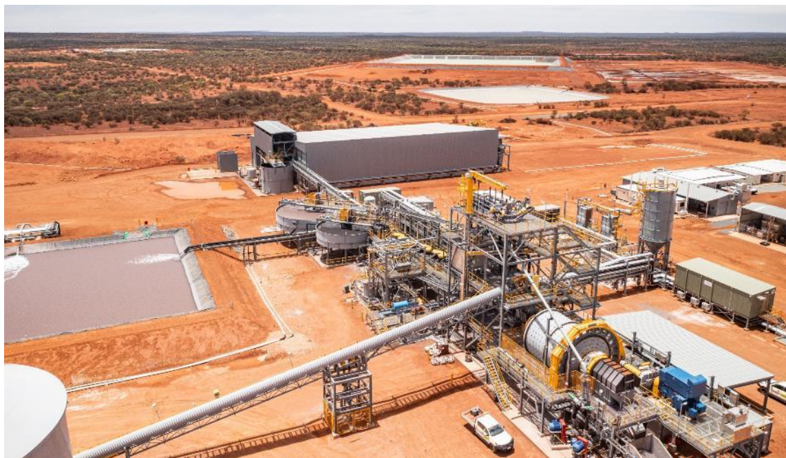
Figure 5 – Processing plant grinding, flotation, thickening and filtration sections commissioned in December quarter (Photo – 20 January 2023).
