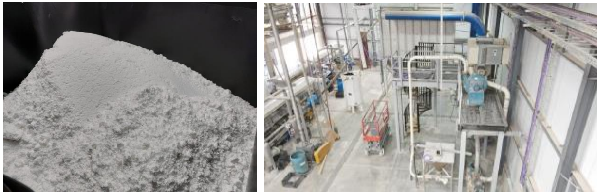
Figures 2-3. Rincon Lithium Project – 2,000tpa Operation Commissioning Works
