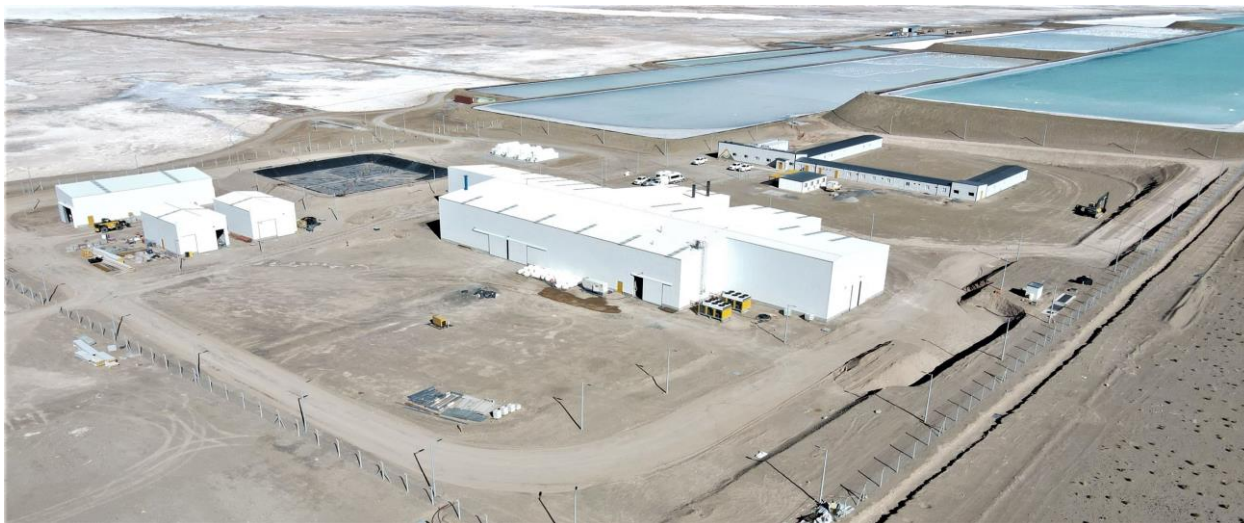
Figure 1. Rincon Lithium Project – 2,000tpa Operation
