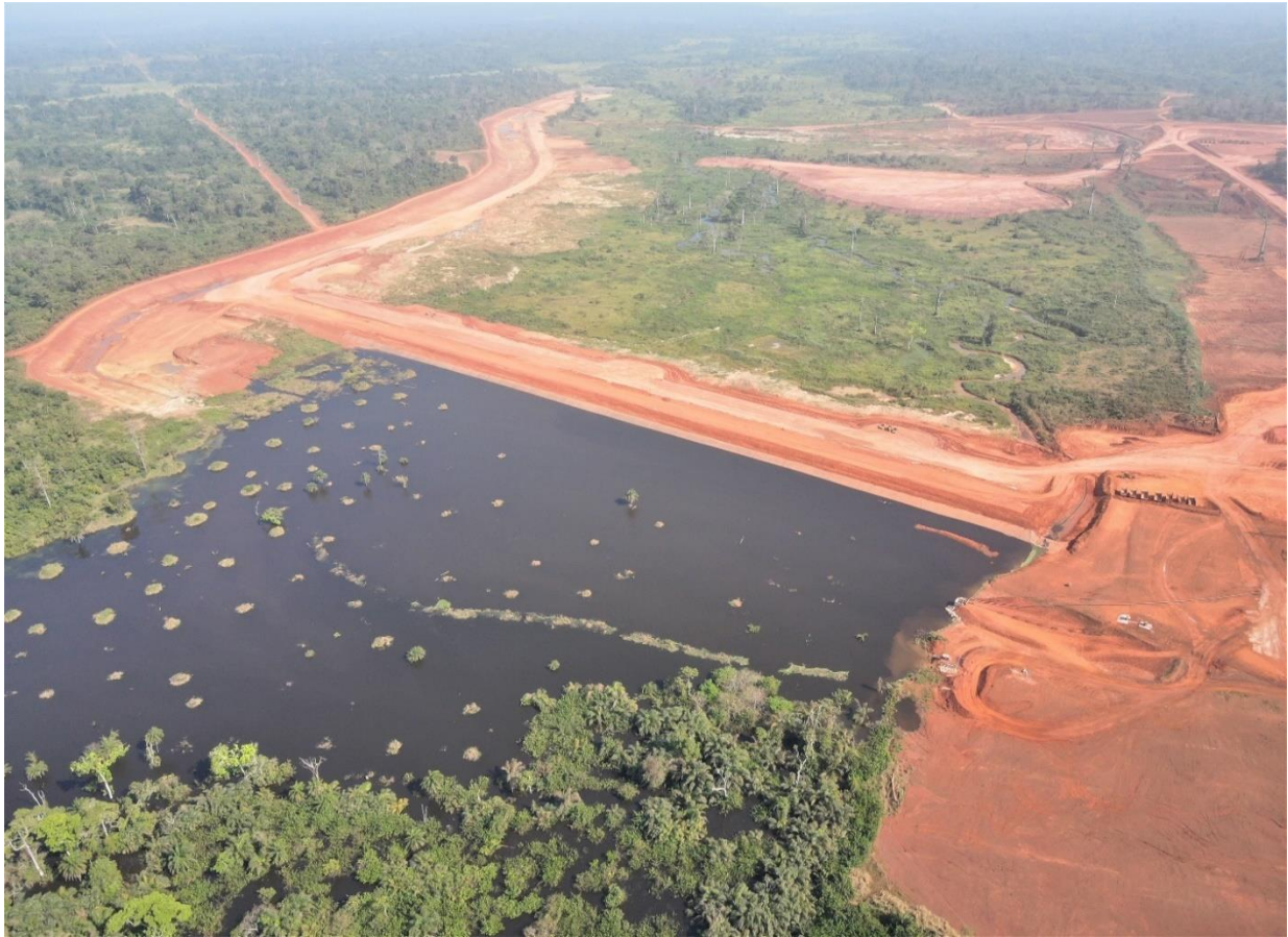
Figure 7: Water storage dam and diversion channel
