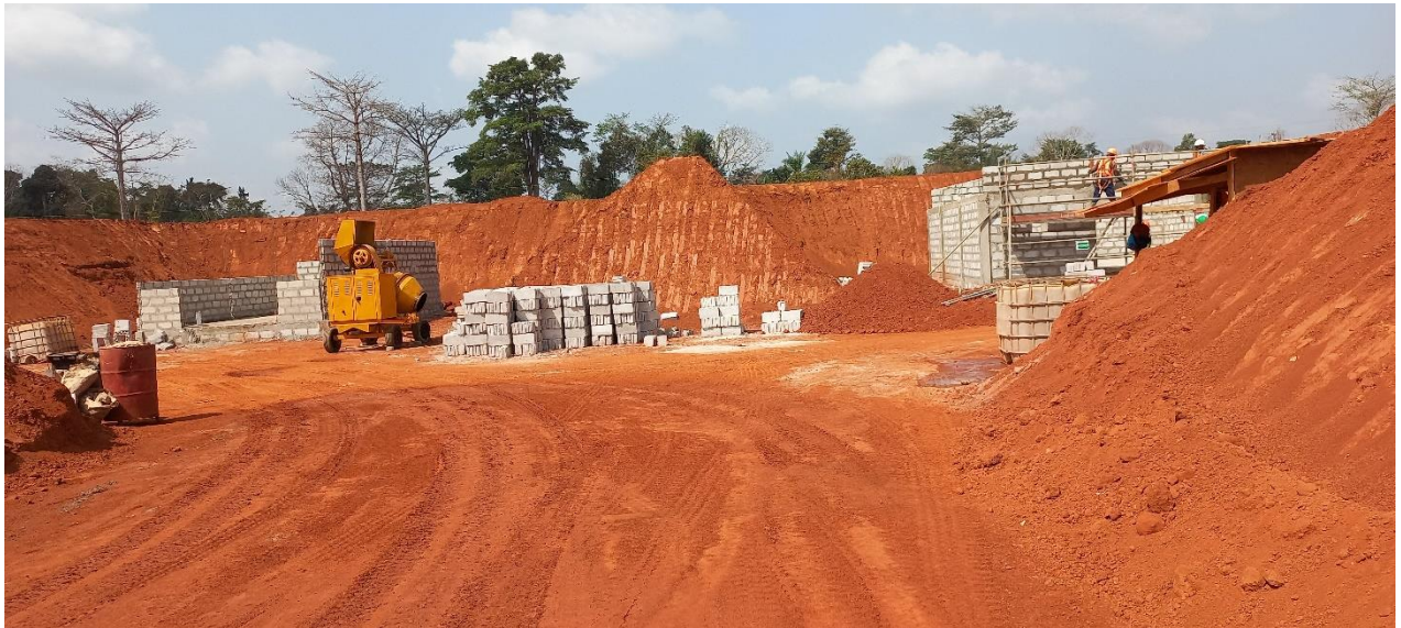
Figure 11: Explosive magazine in construction in early January 2023
