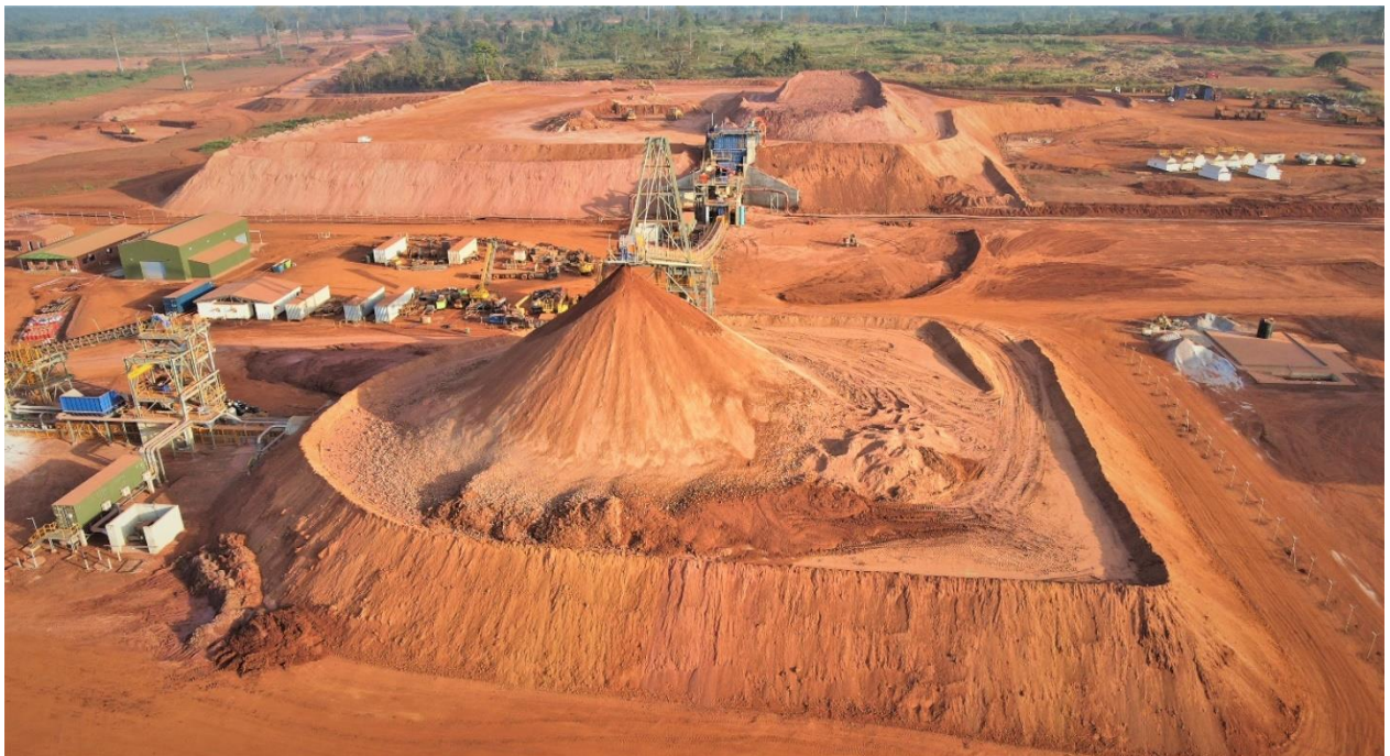
Figure 5: ROM, Crusher, CV-01 and Reclaim
