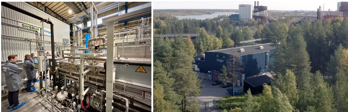
Figure 2 Kiln in Main Hall (L) of Talga’s Electric Vehicle Anode plant in Luleå, Sweden (R).
