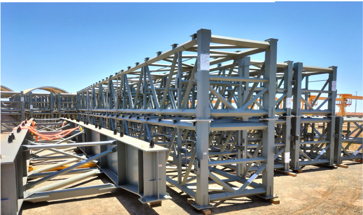
Figure 2: Jetty Structural Steel - Dampier
