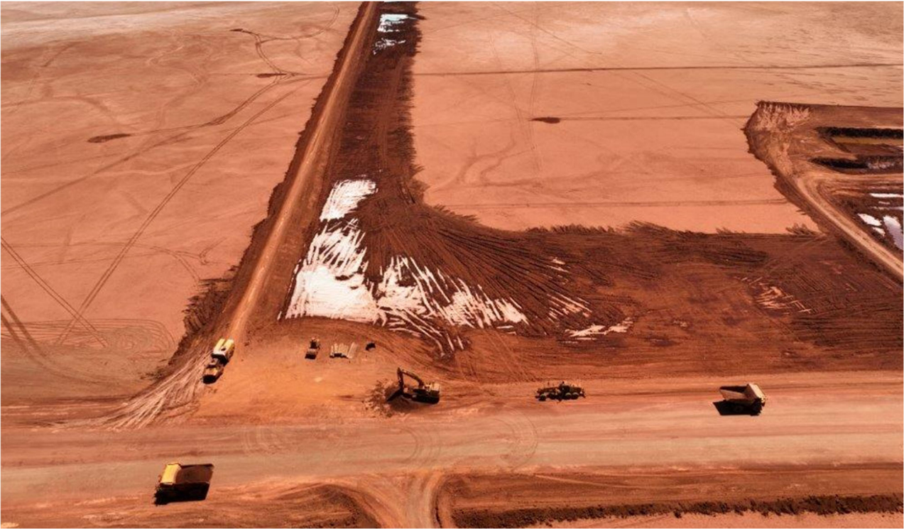
Figure 3: Pond 3 levee construction
