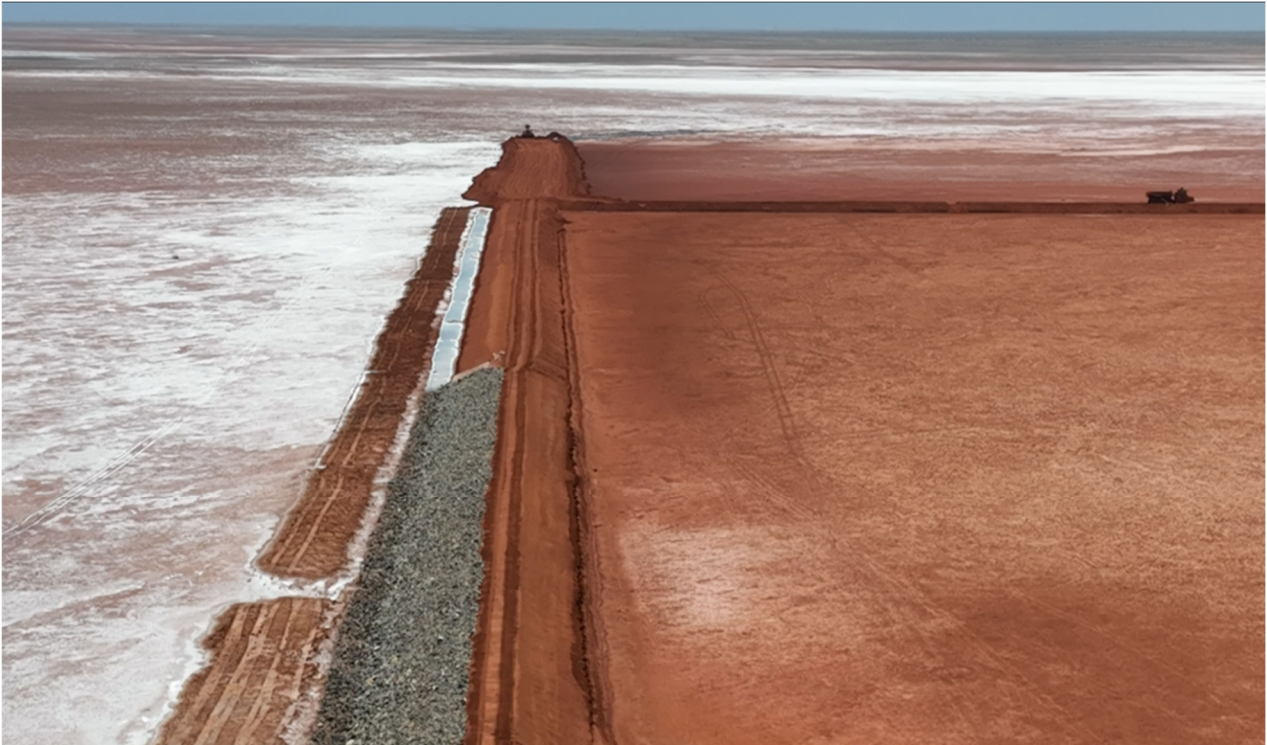
Figure 1: Pond 5 & Trial Embankment tie in
