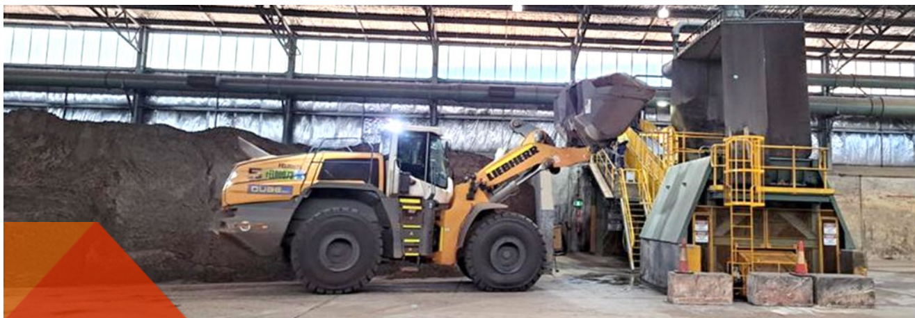
Figure 2 Coburn Project – First Load of HMC at Berth 4 Port of Geraldton WA, (December 2022)
