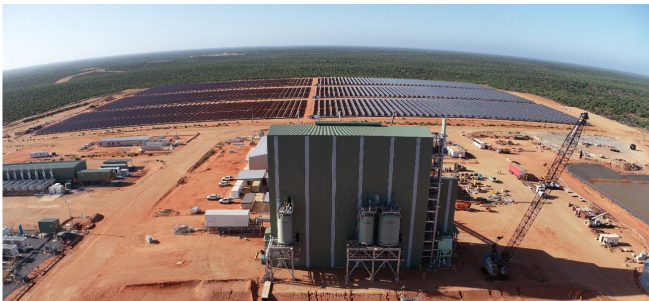
Figure 6 Coburn Project – MSP Construction Complete and Commissioning Underway
