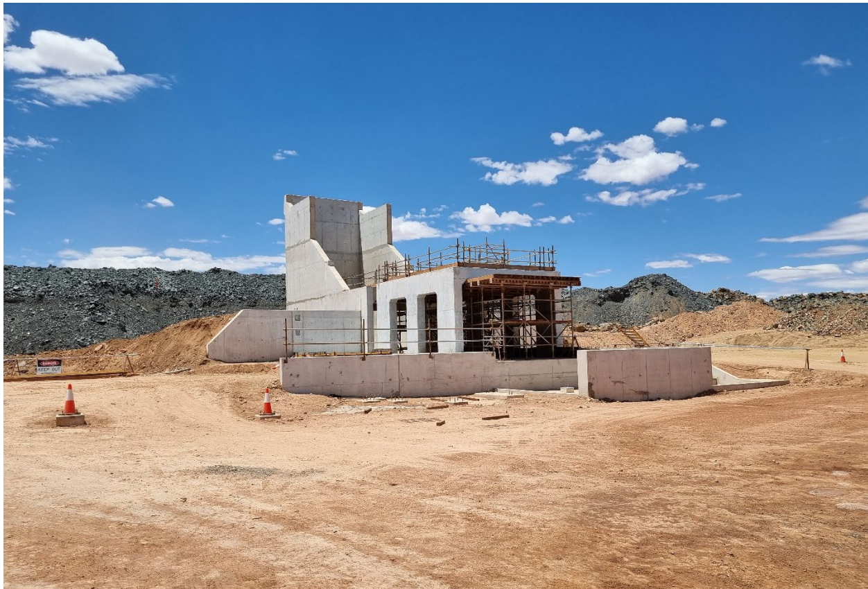
Figure 3: Construction progress on the ball mill foundations at the processing plant as at 24 January 2023
