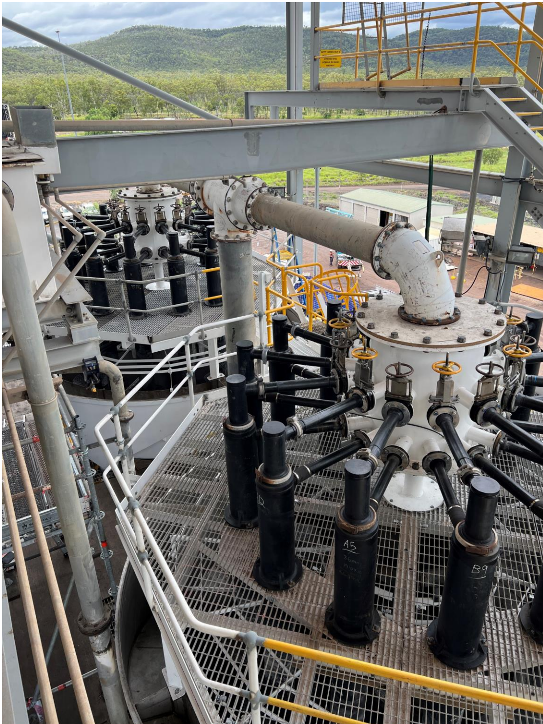
Figure 3. Refurbished floatation cells refitted in the Burton CHPP
