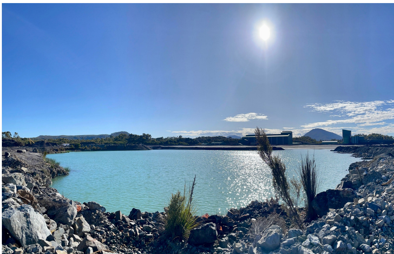
Figure 9. Avebury decant pond with tailings beach and processing plant in background.
