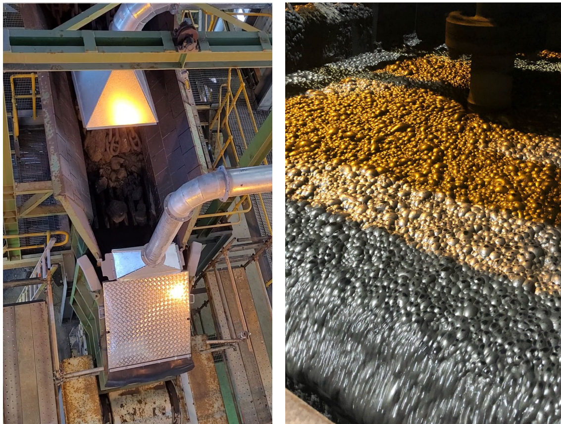
Figure 4. Dust extraction system over primary crusher (L) and concentrate in float circuit (R).
