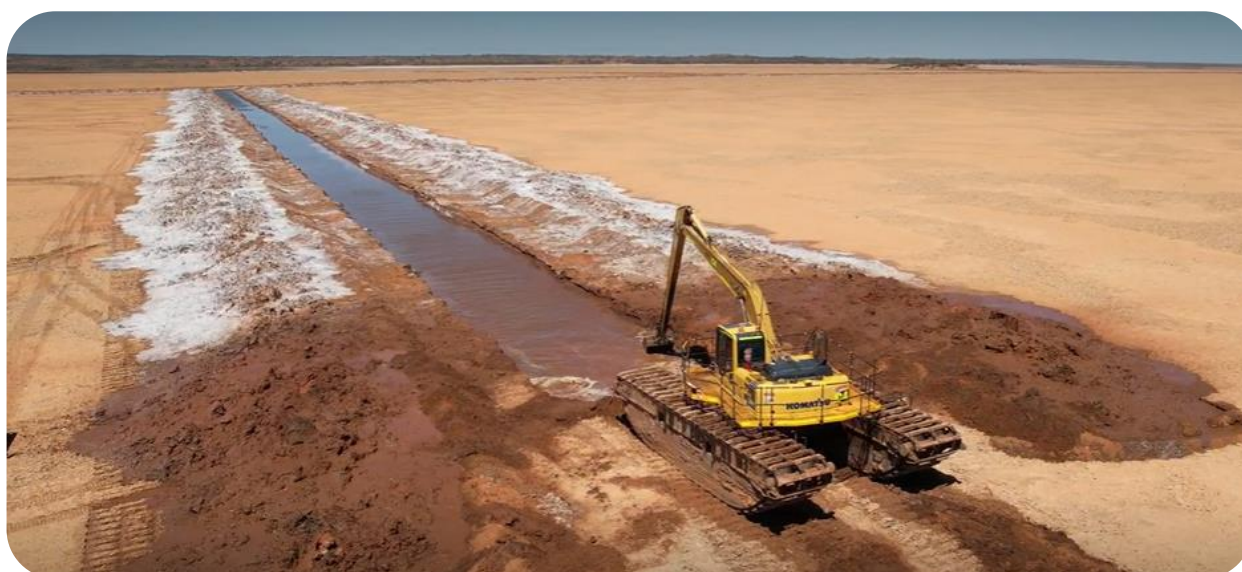
Lake Sunshine trenching operations, October 2022
