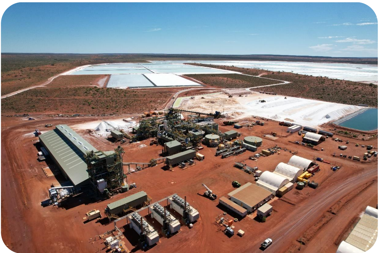
Beyondie SOP plant and evaporation ponds, November 2022.
