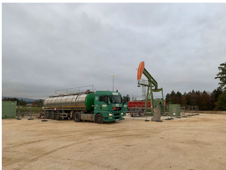
Oil tanker offloading at Anshof-3 location
