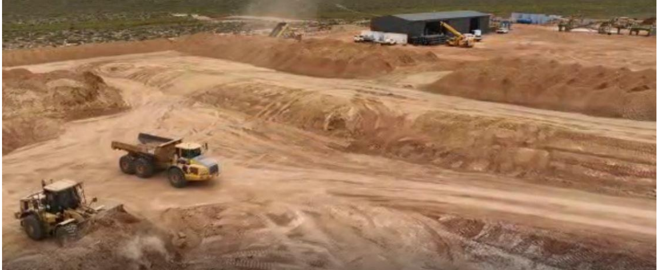
Figure 1 & 2: TSF area being cleared
