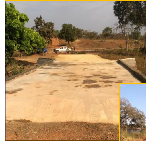
Bridge repair into Kobada village
