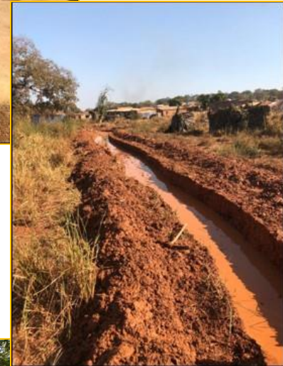
Drainage channel construction around main village
