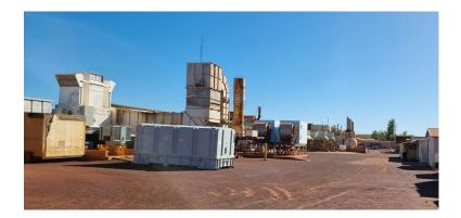
Nifty generates its own power from a gas fired captive General Electric 21MW power plant. Nifty also has on standby two 2.5MW gas / diesel turbine generator sets, two 2MW diesel generator sets and two 1MW diesel generator sets.
