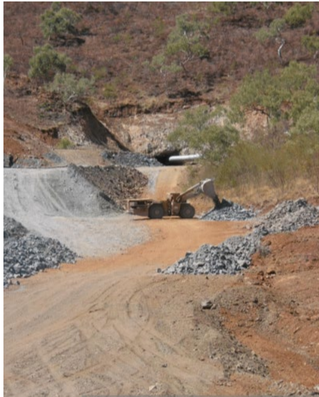
Portal decline during stoping trial, 2002.
