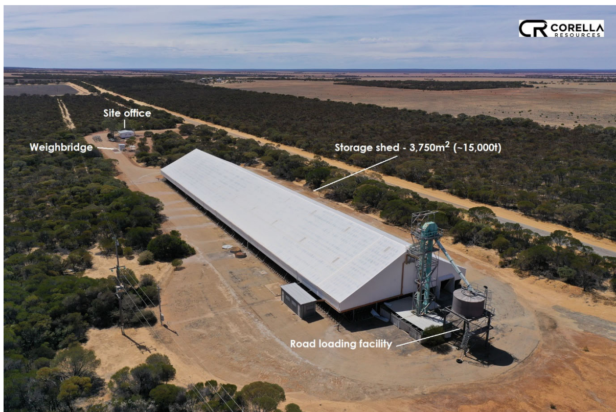
Figure 1 Tampu storage facility (view looking NNE)
