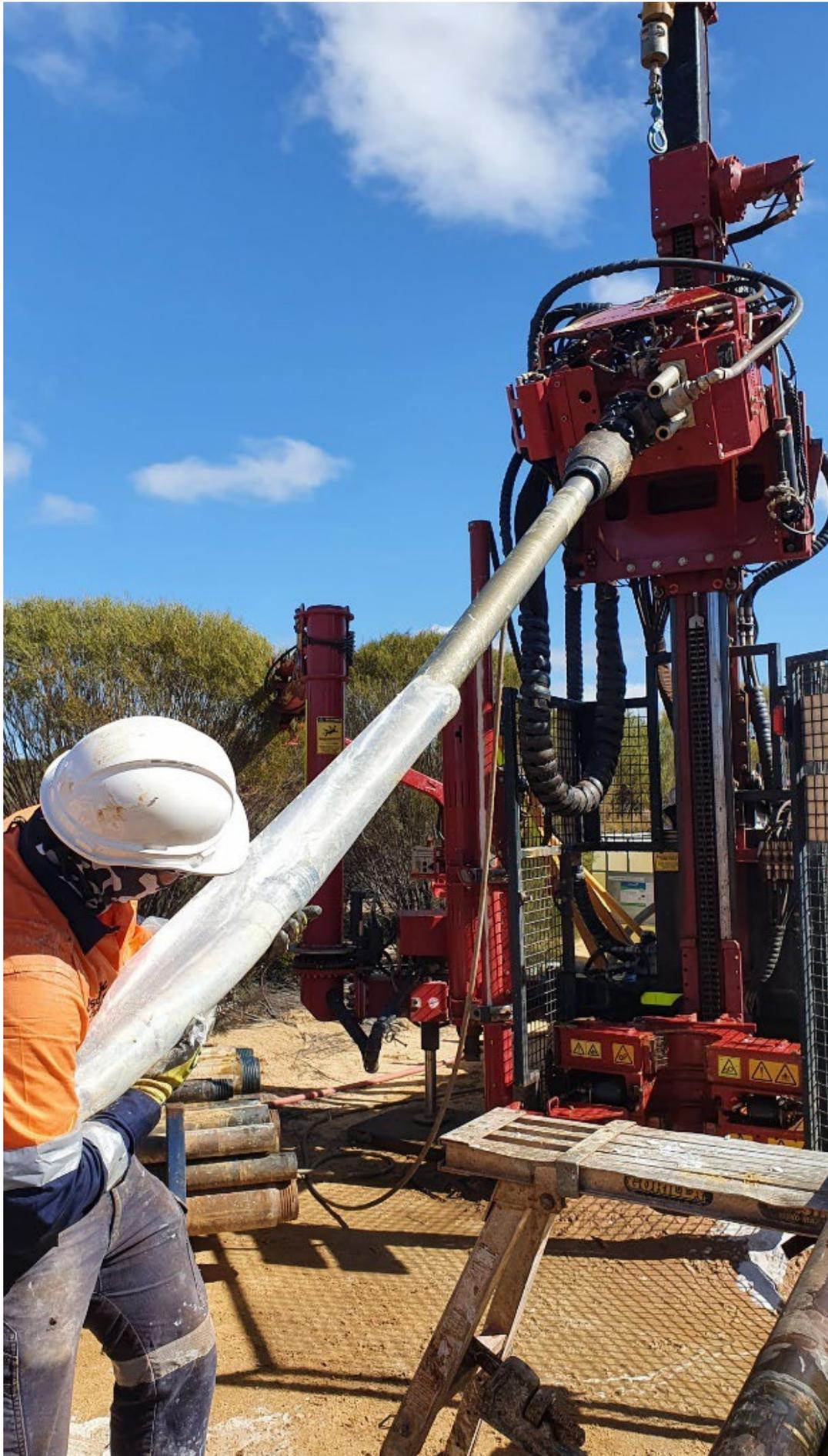
Figure 5: 2022 Resource Definition Sonic drilling at Tampu
