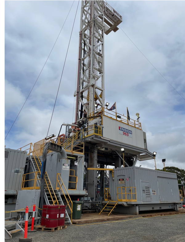
Ensign 965 rig under contract to large regional operator
