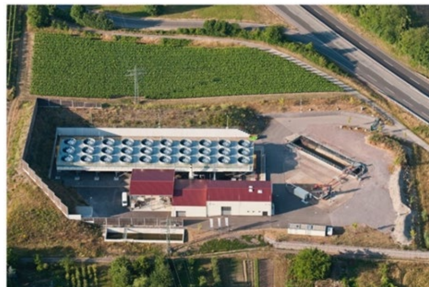
Vulcan's existing Insheim ORC plant
