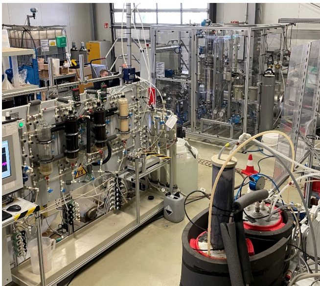
Pilot Plant Low Pressure (LP)
