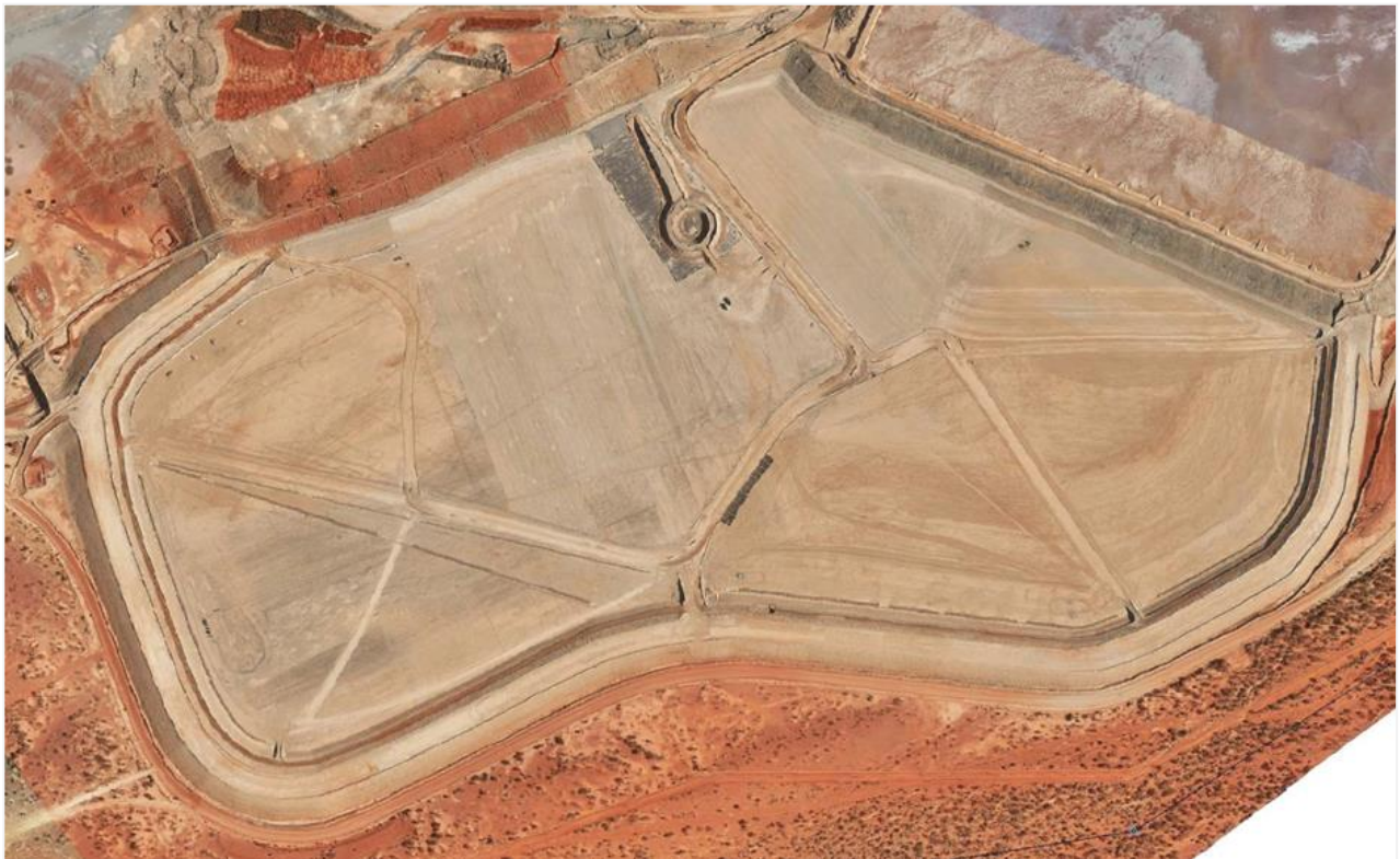
Figure 2: TSF5 is on track for commissioning in early April 2023.
