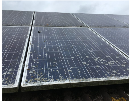
Algae and Lichen build up on solar panels 3
