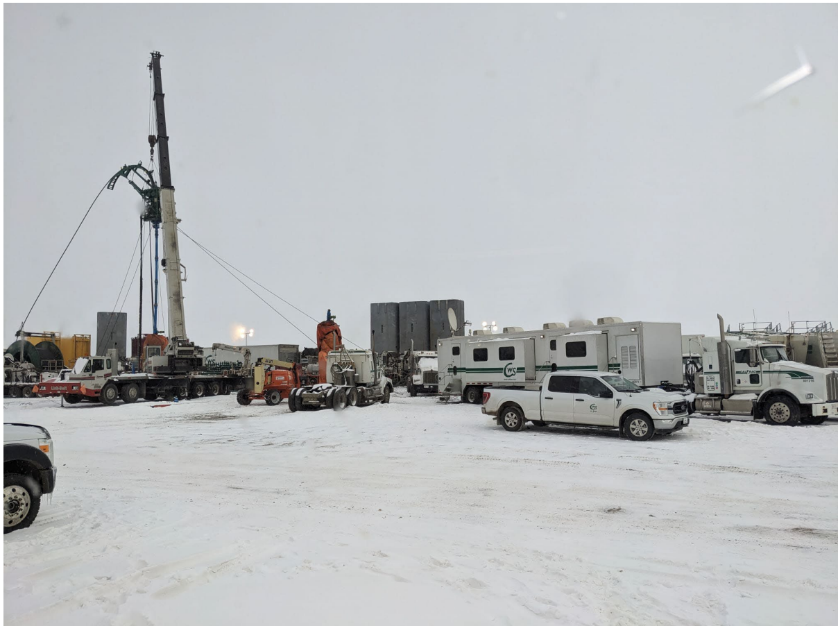
Figure 3: Frac'ing operation on Pisces #8 & #9 pad
