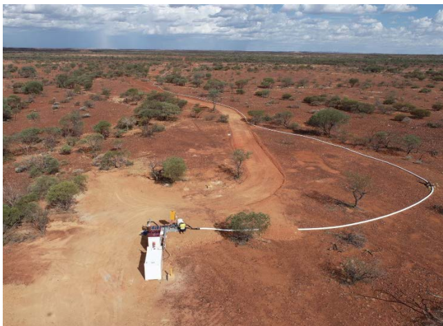
Figure. 3 SipHon borefield in operation
