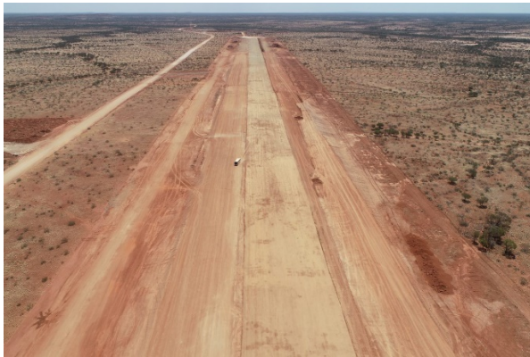
Figure. 1 Mine Site Airstrip: nearing completion and first operations.
