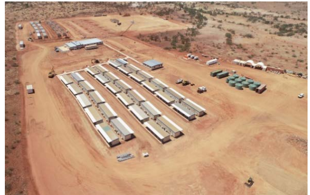
Figure. 2 Kurbilli Accommodation Village: Phase 1 and 2 taking shape.
