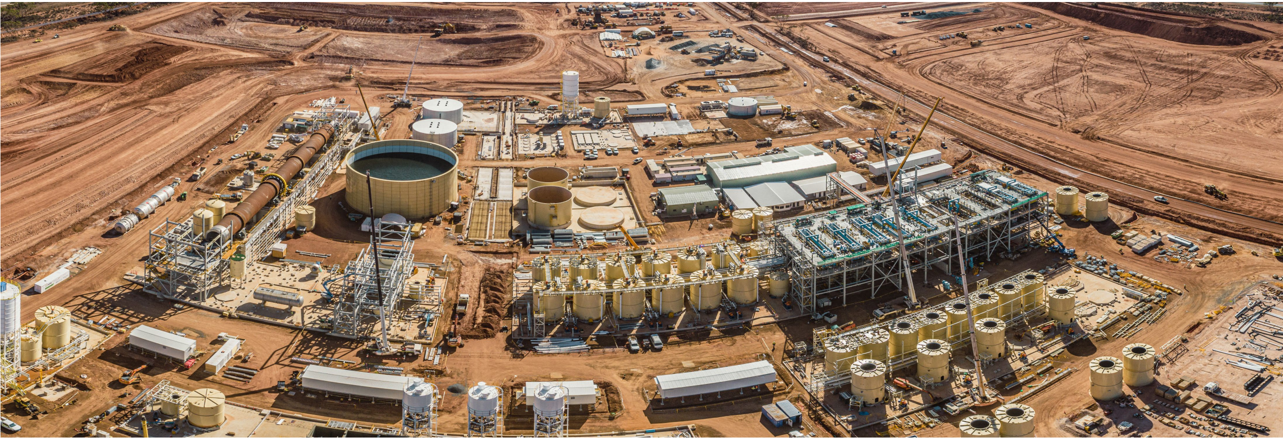
Panoramic photo of Kalgoorlie Rare Earths Processing Facility
