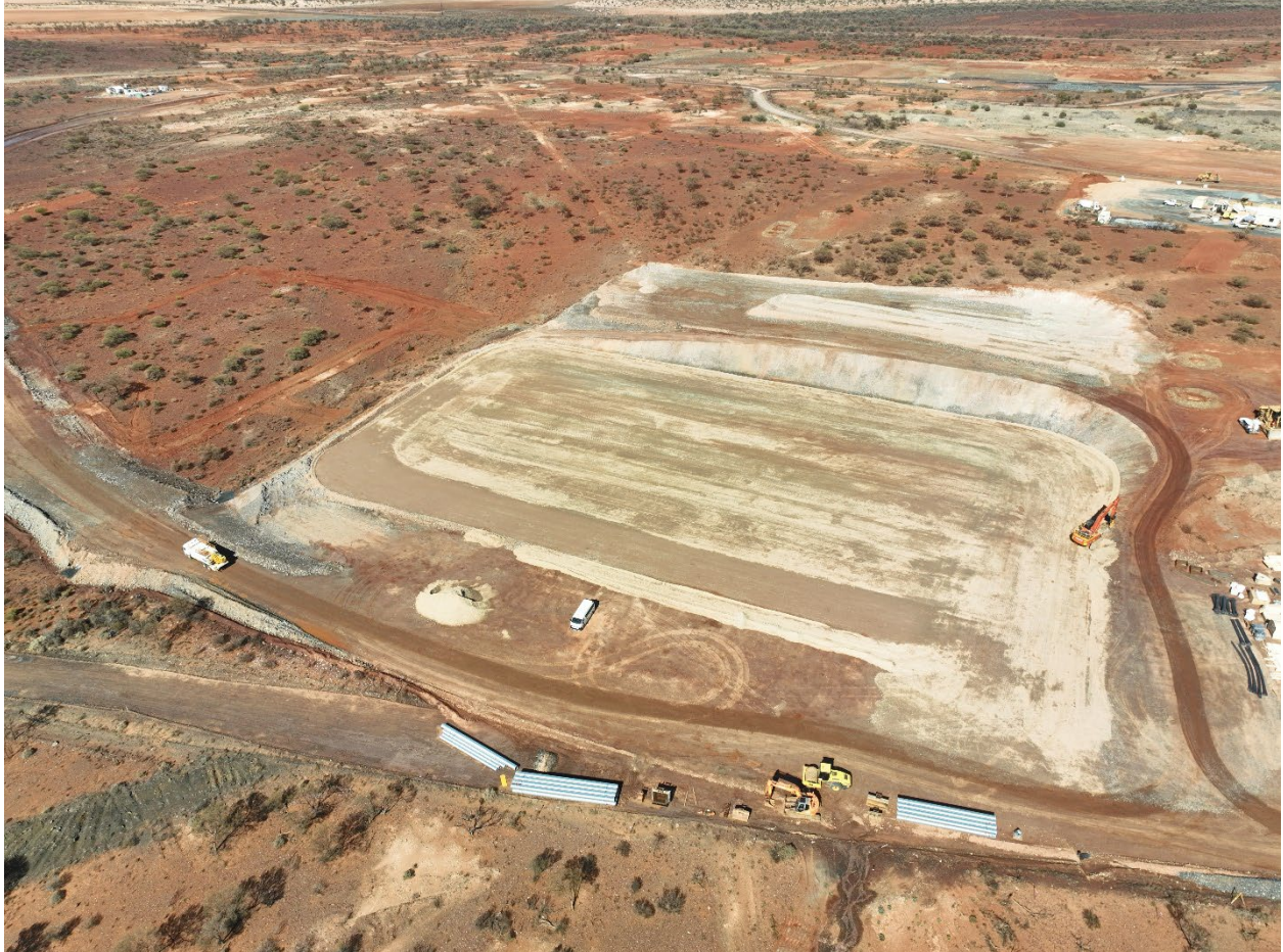
Figure 9: Bulk earthworks complete for thermal power station and battery pads. Concrete works to start later this quarter.
