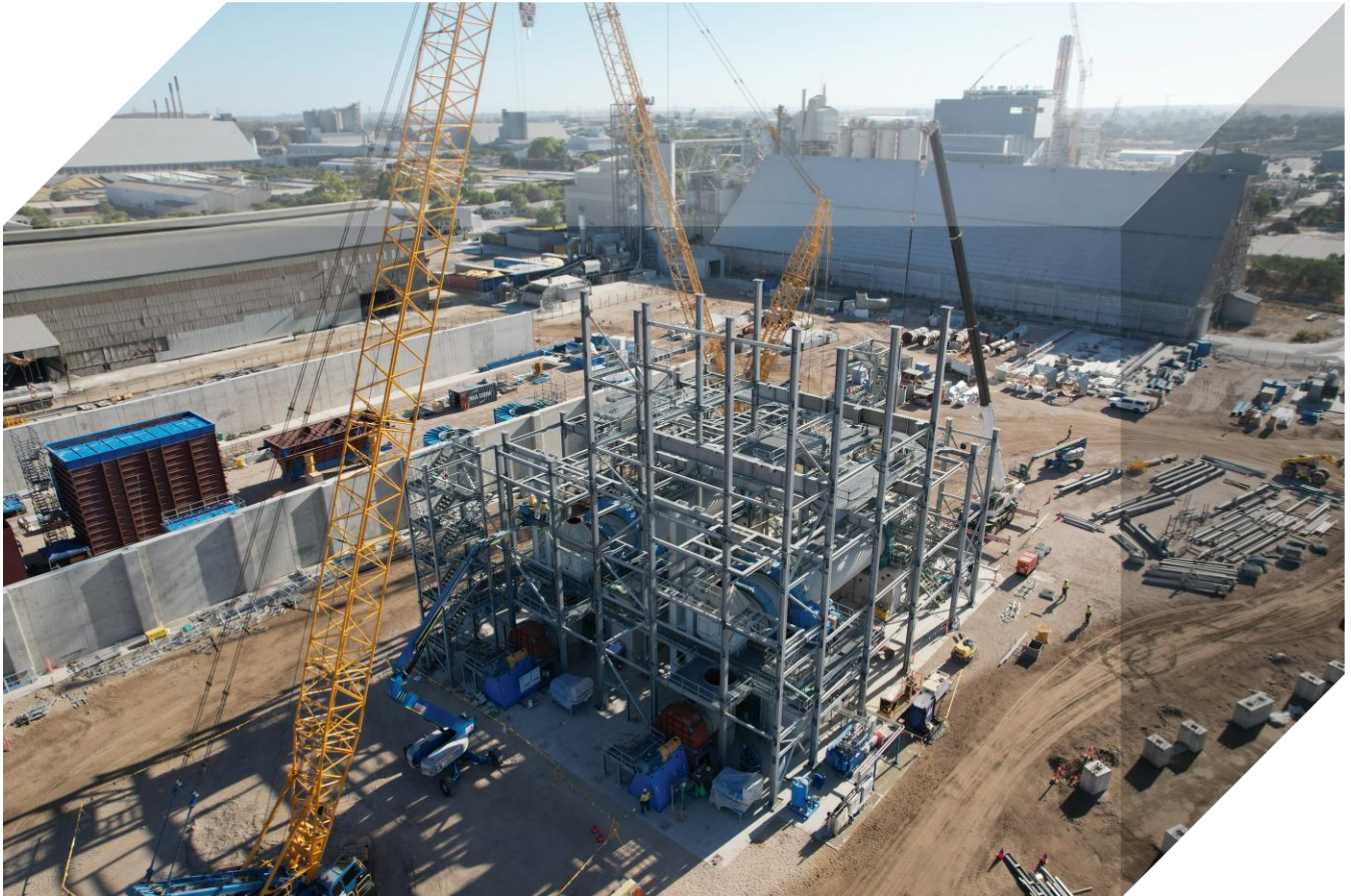
Image: Cockburn Cement Kwinana Upgrade Project (SIMPEC)
