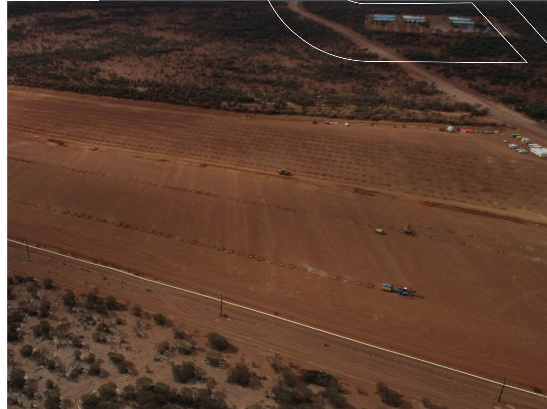
Installation of 9MW solar farm (Duketon)
