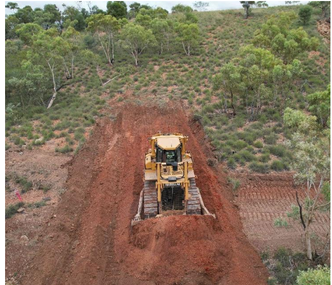
Figure 2. Clearing drill pads at Lady Tresca ready for drilling
