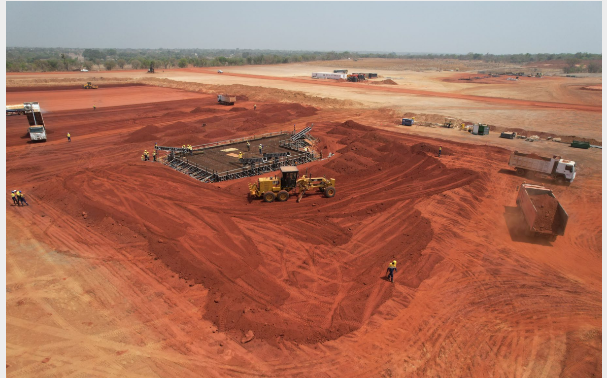
Earthworks in mill area construction offices in background
