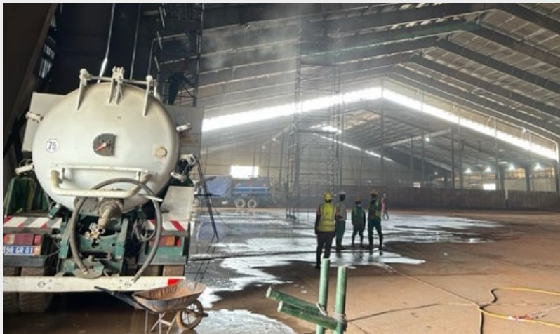
Shed cleaning in readiness for DSO
