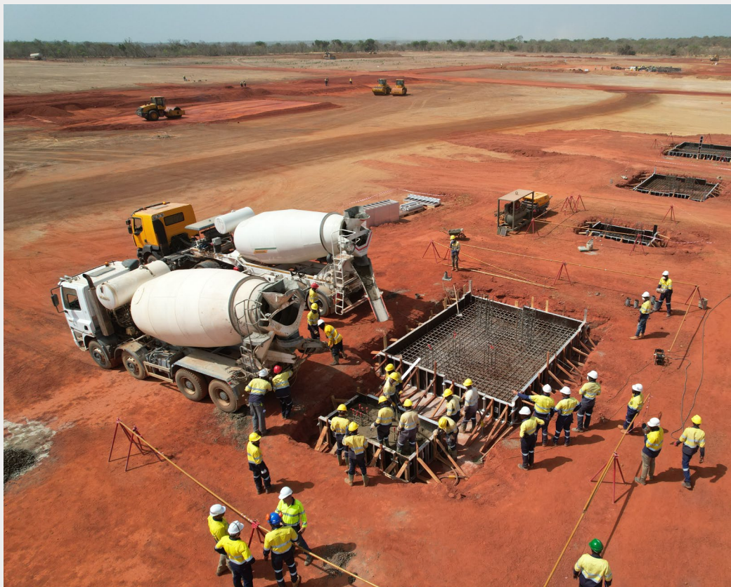
Crushing conveyor footings being poured First concrete pour on 14 Feb
