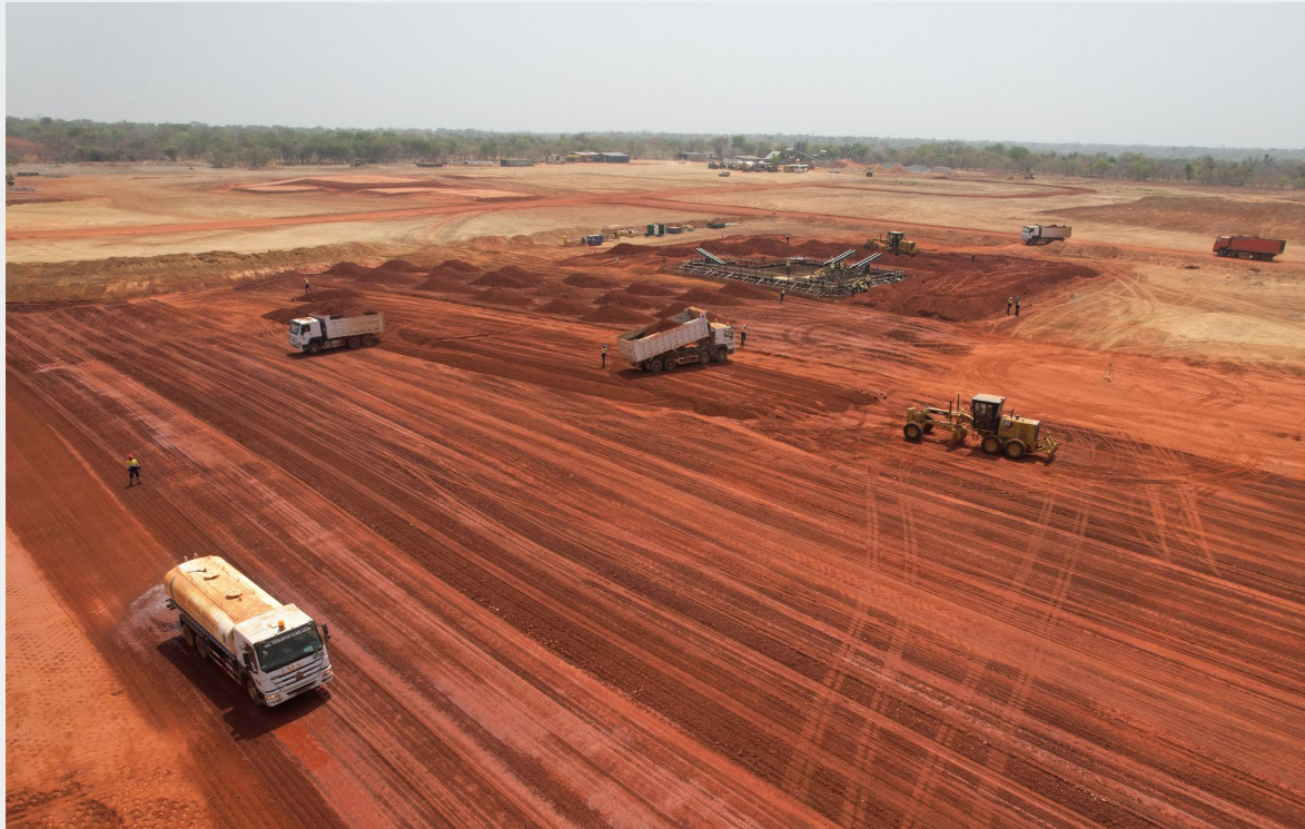
Process plant site: clay removal and backfill Next: prepare foundations of mag circuit and thickeners
