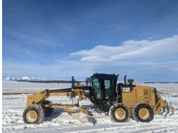
Figure 5: Jesse-2 well pad construction begins in Utah
