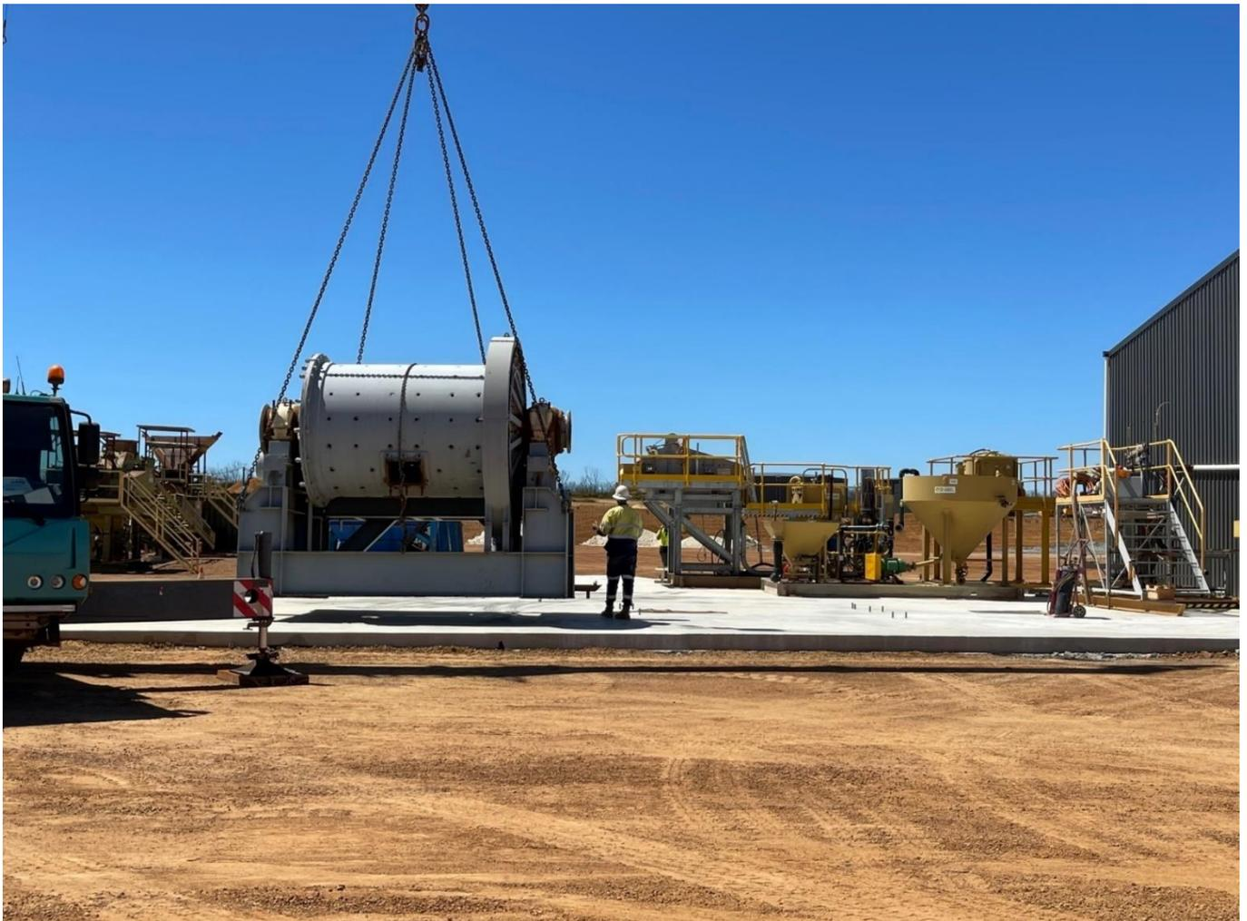
Figure 6: Trommel frame being placed on foundation.
