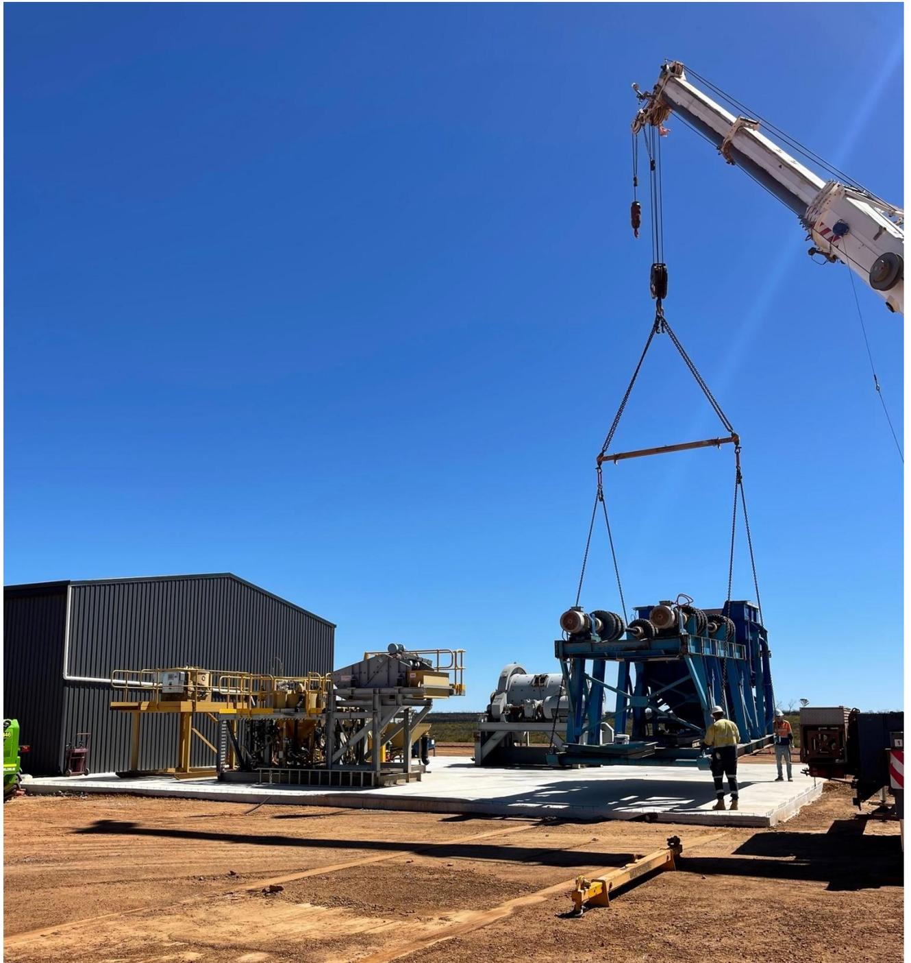
Figure 7: Trommel being assembled on foundation.
