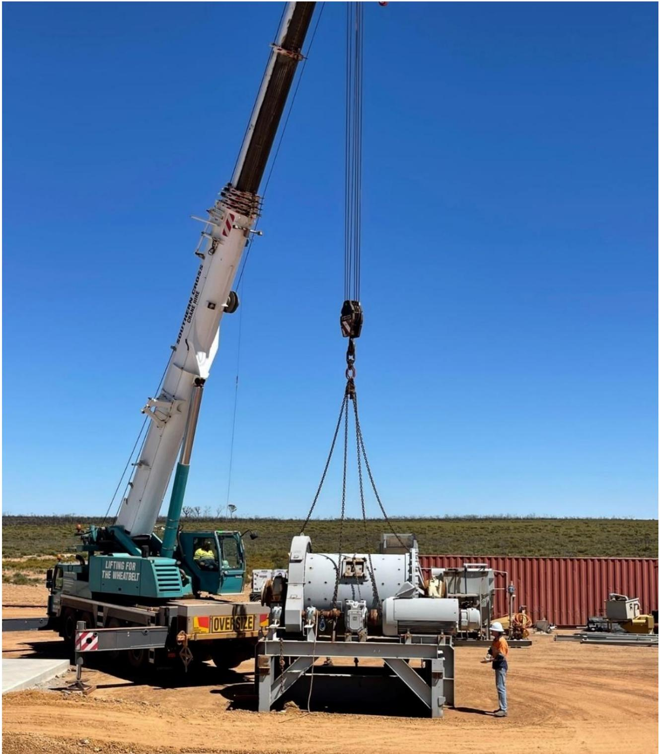
**Figure 5: Ball mill being placed on foundation**
