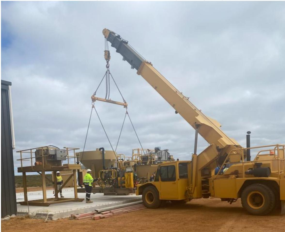
**Figure 2 & 3: Spinner being placed on foundation at Kat Gap Processing Facility.**
