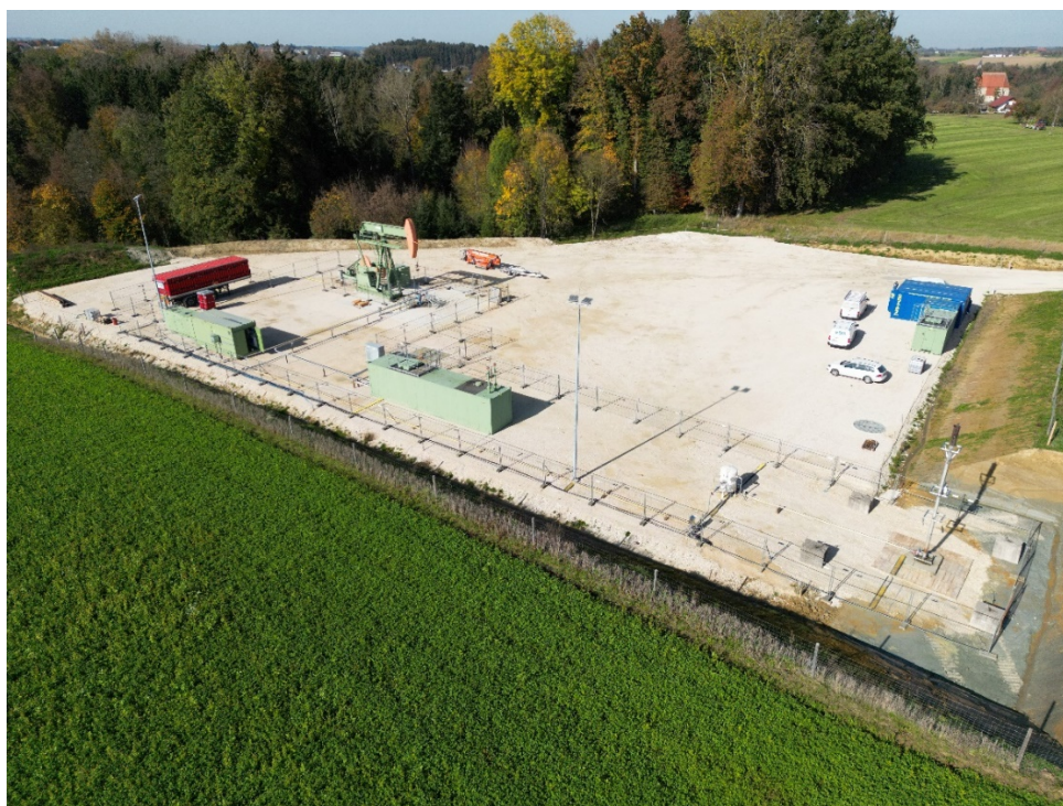
Figure 2: The Anshof-3 well and early production unit
