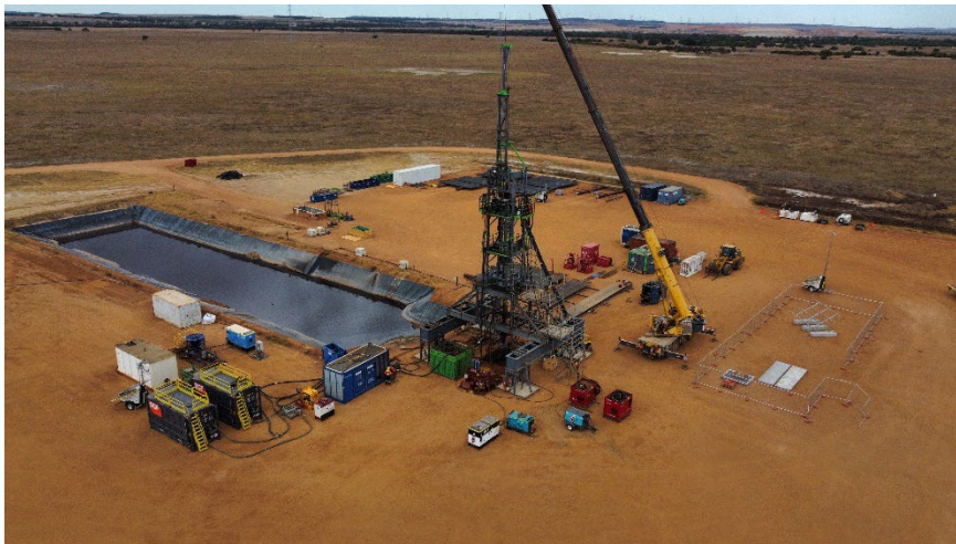
Production completion installation with a workover rig at Walyering-5
