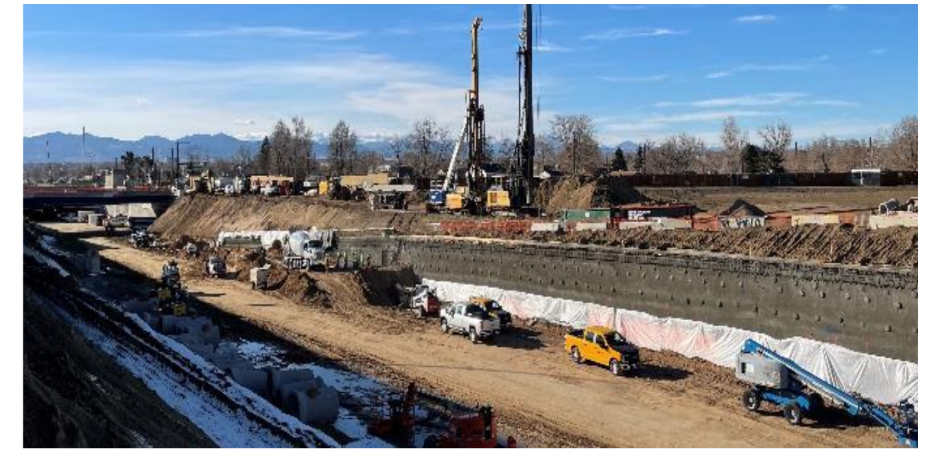
I-70 Shotcrete project in Denver
