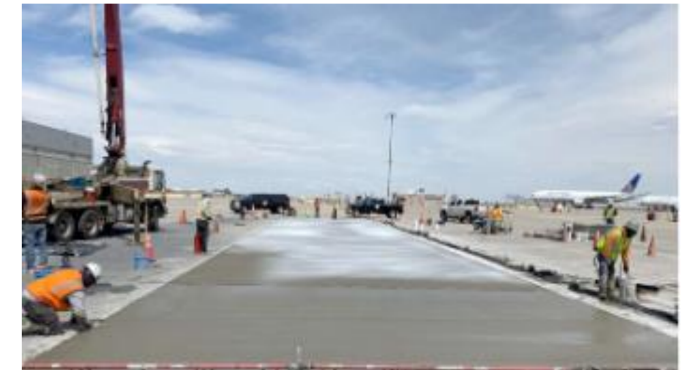
Denver Airport- concrete replacement -United Airlines
