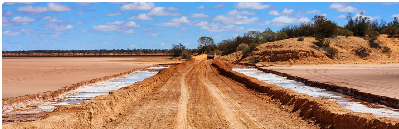
FIGURE 2: CAUSEWAY ACROSS LAKE SURFACE TO FACILITATE DRILLING CAMPAIGN
