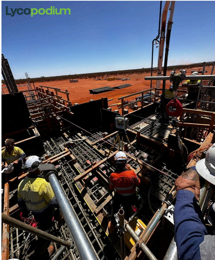
Foundation for the SAG Mill well advanced
