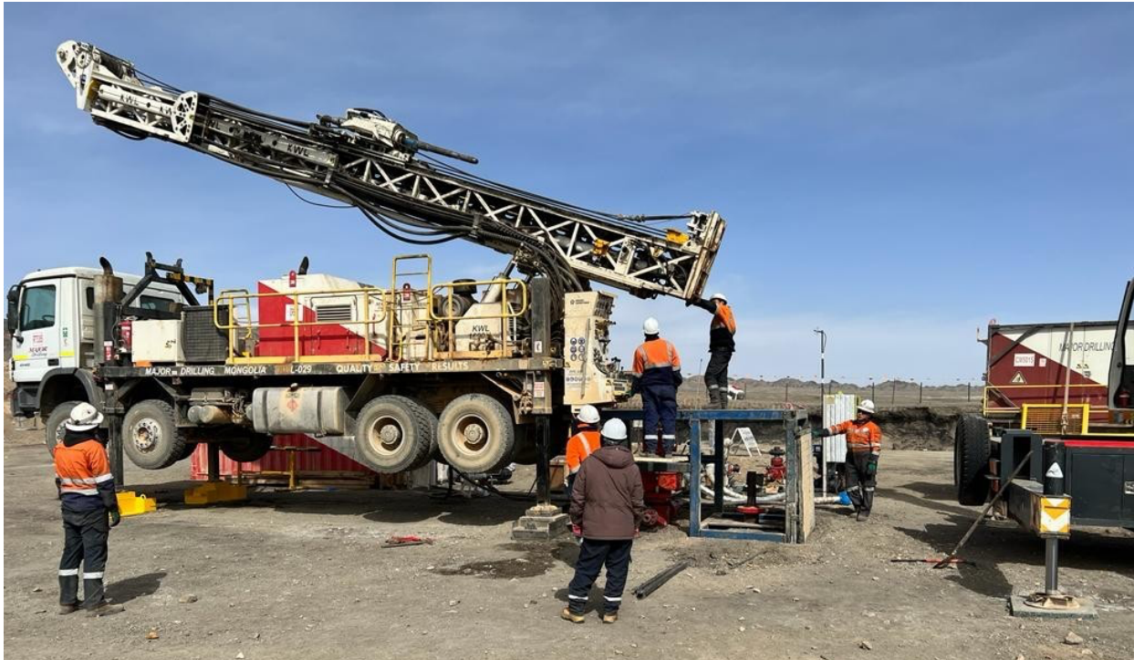
Major Rig setting up for routine workover operations and Nomgon-8
