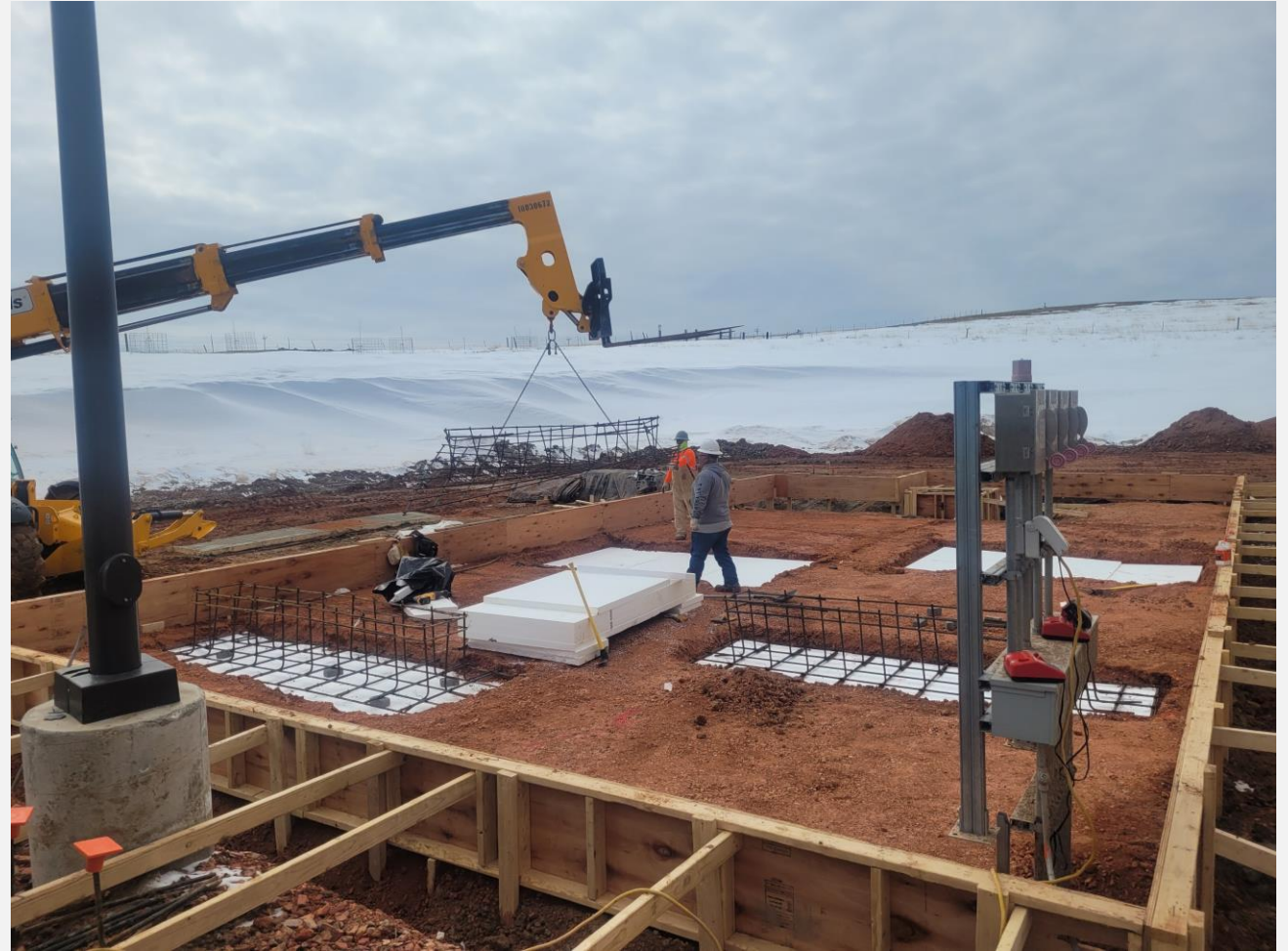
March 2023 Chemical Storage System Construction
