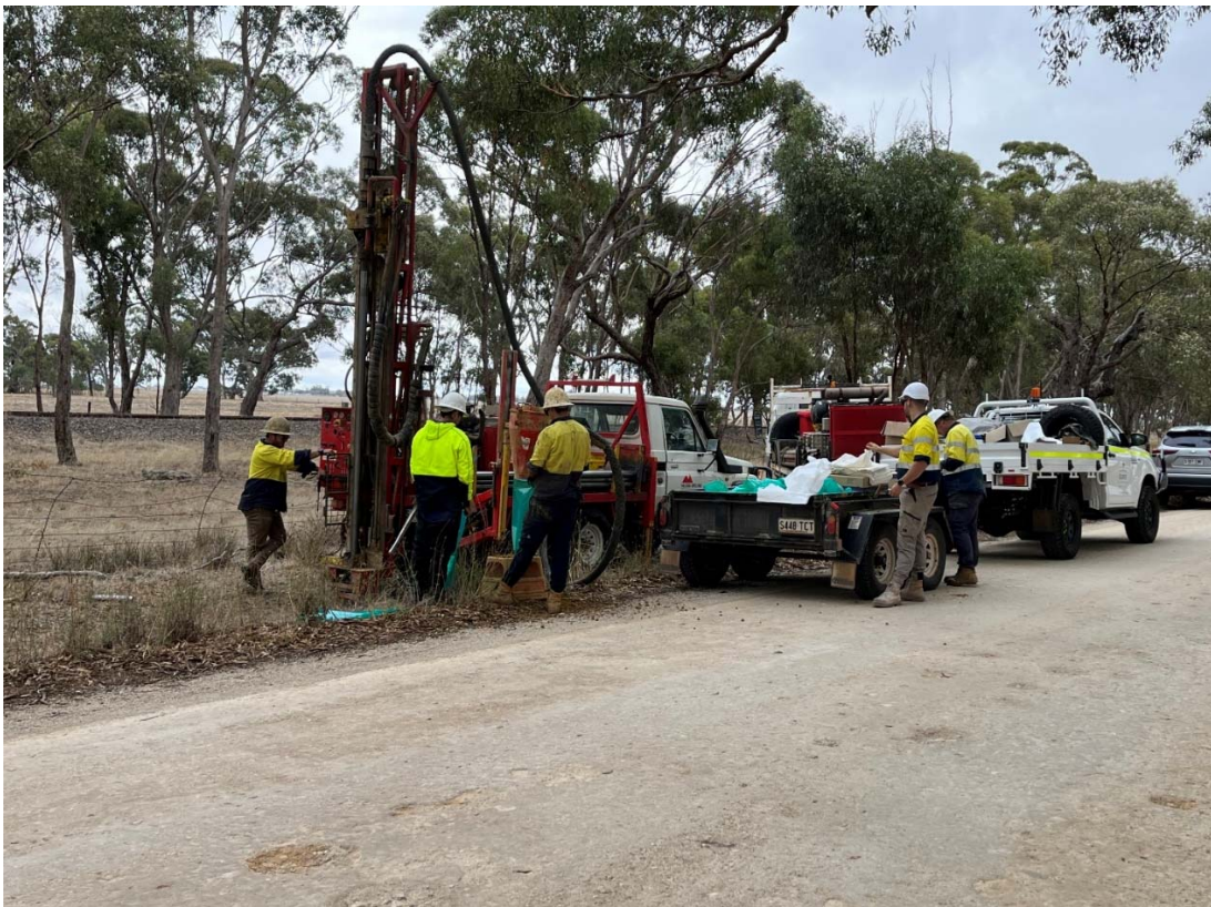
Image 1: Roadside Drilling Team on Bangham Road south of Bordertown
