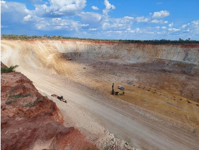
Figure 1: Drilling continues at Anthill ready for next blast
