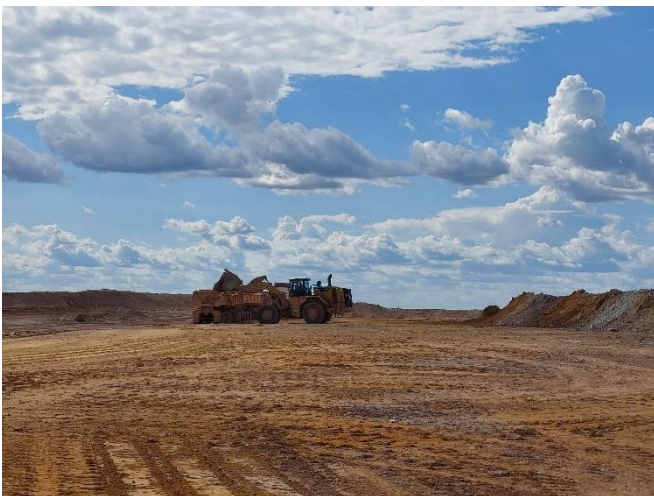
Figure 3: Stockpiling at Anthill ROM Pad continues
