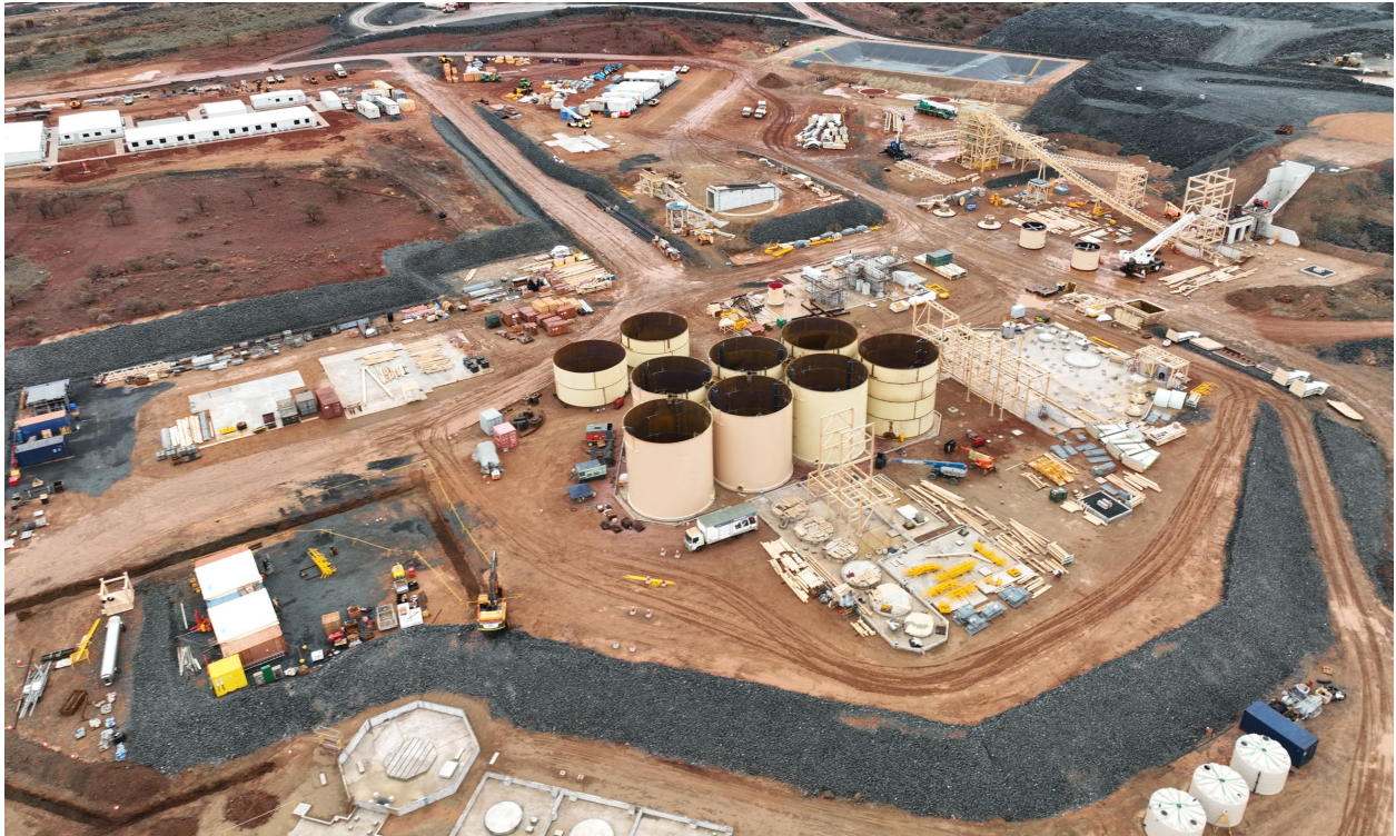
Figure 4: Processing plant works as at 31 March 2023, with critical path CIL tank construction prominent in the centre with tank painting commencing.
