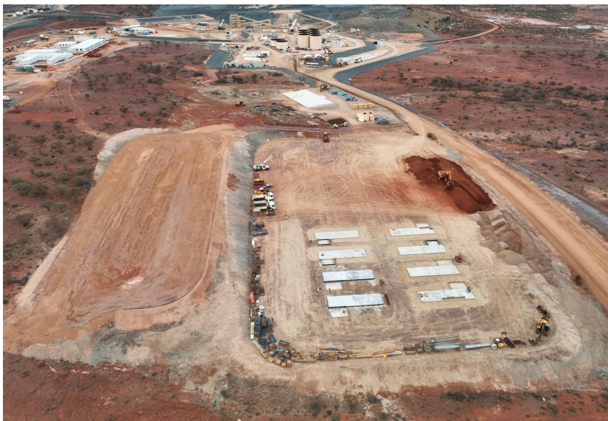
Figure 6: Power station construction including commencement of structural concrete for thermal generators.
