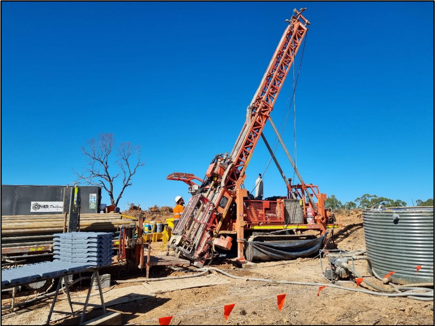
Figure 1 – Wisemans Creek -Phase 2 drilling, diamond drill set up on first hole
