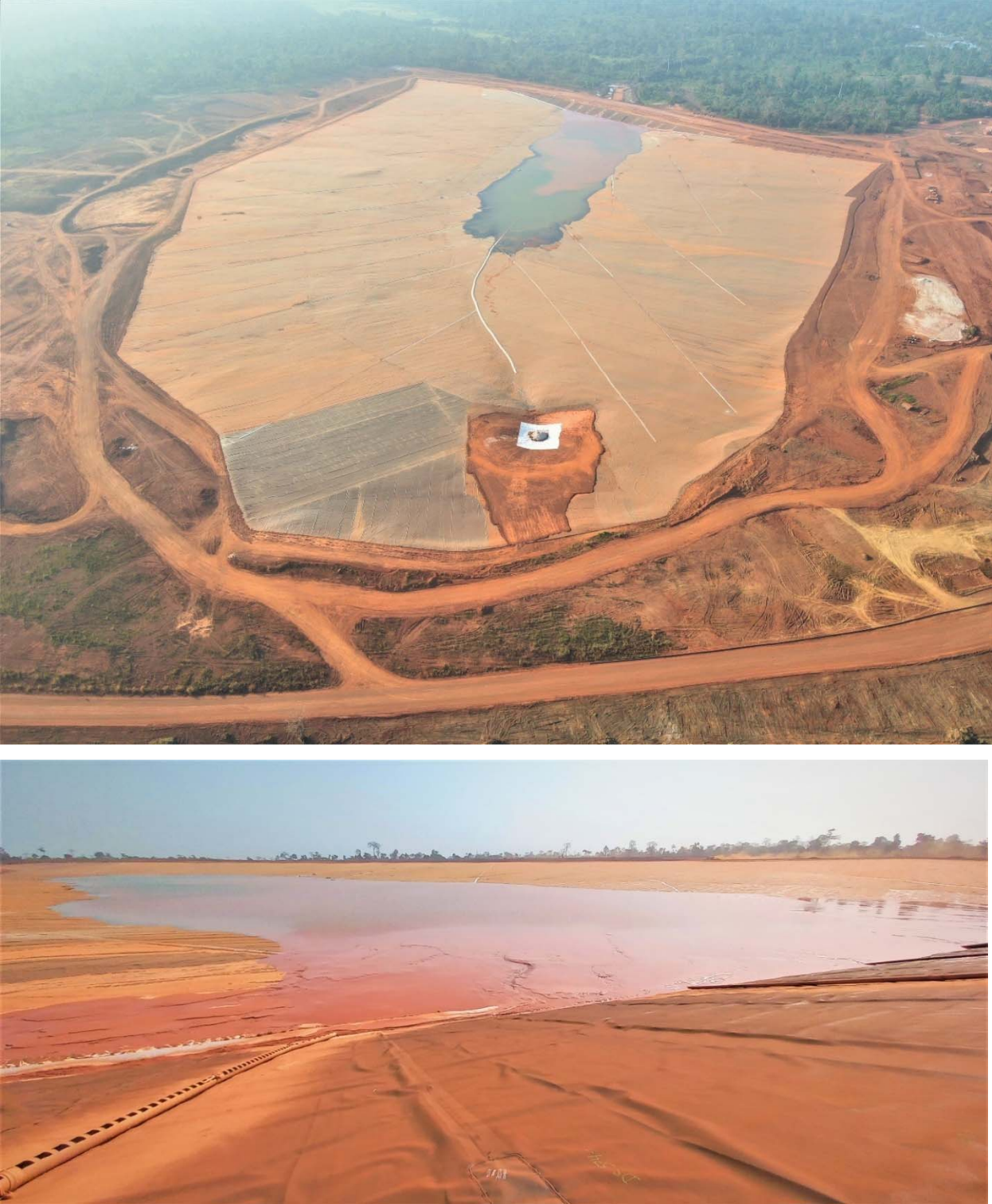
Figure 6: Tailings Storage Facility (TSF) at the beginning of January 2023
