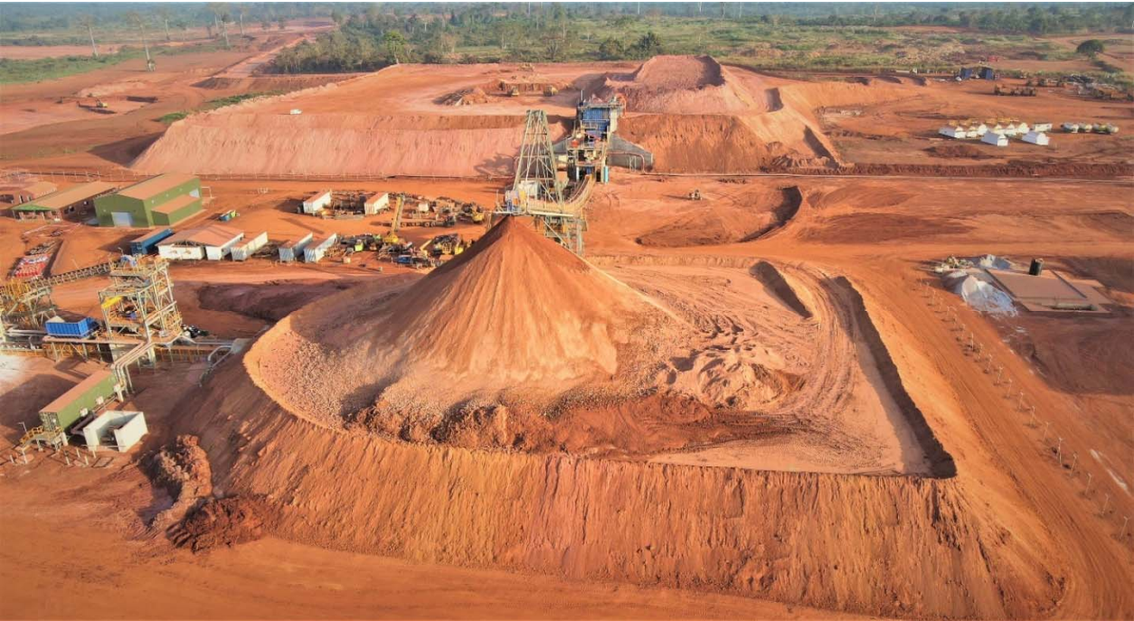
Figure 5: ROM, Crusher, CV-01 and Reclaim
