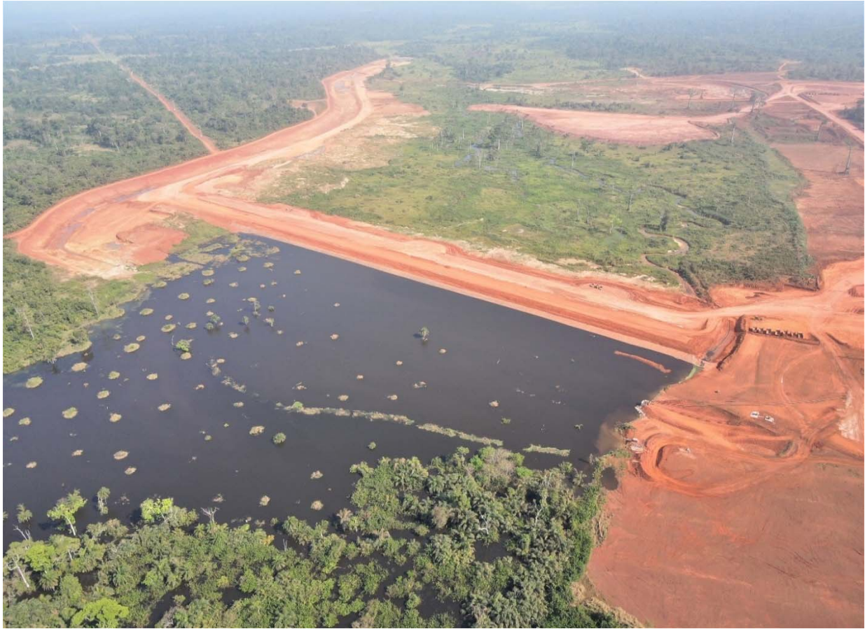
Figure 7: Water storage dam and diversion channel
