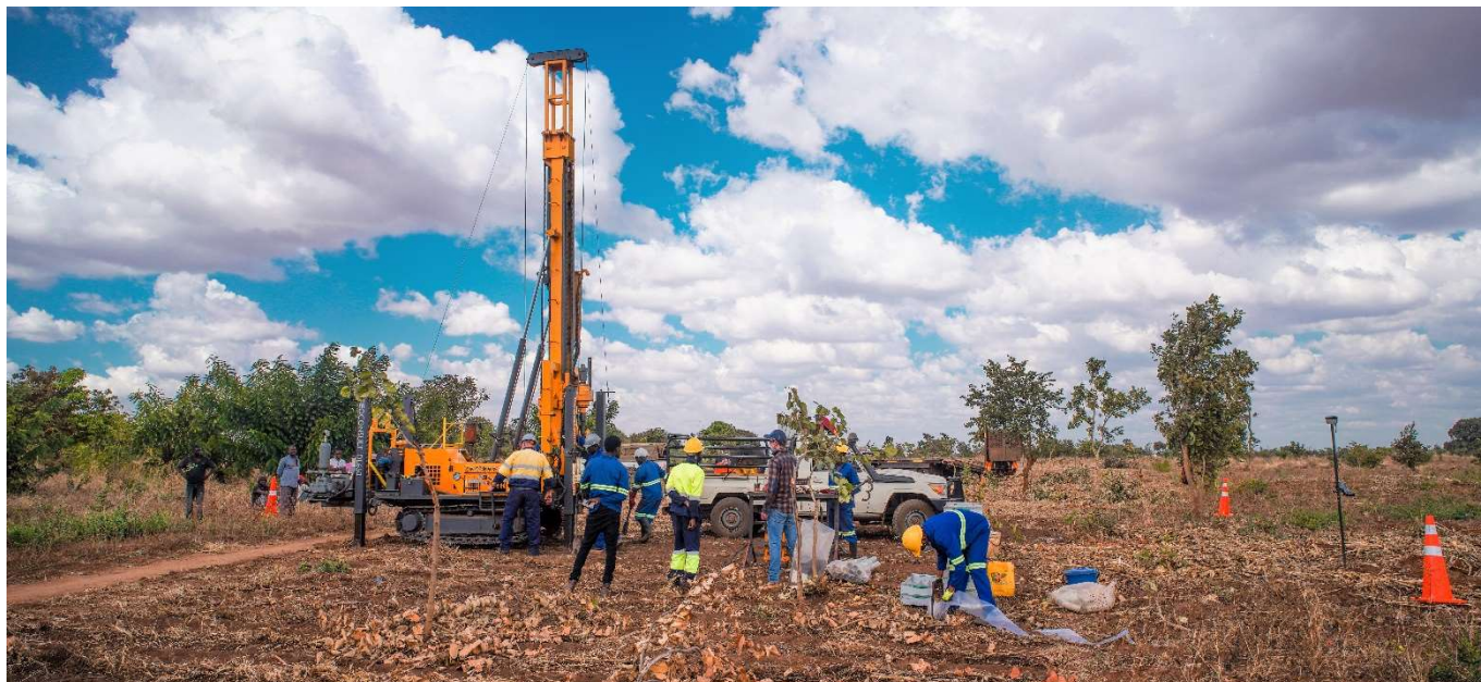
Figure 9: Core drilling (push tube) in action at Kasiya
